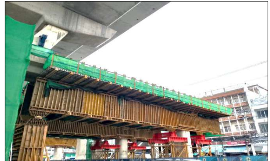
Install Steel Crossheads Pier Type YT-1 MLP04-17
