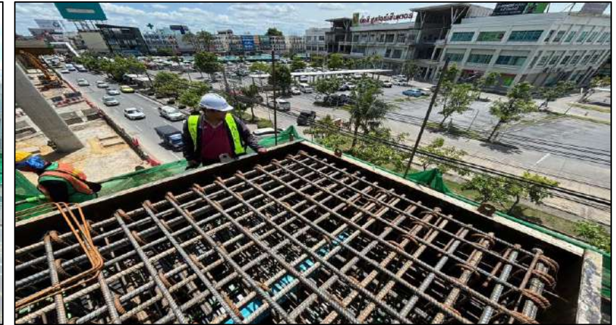
Install Steel Crossheads Pier Type P-1 ROF2-22
