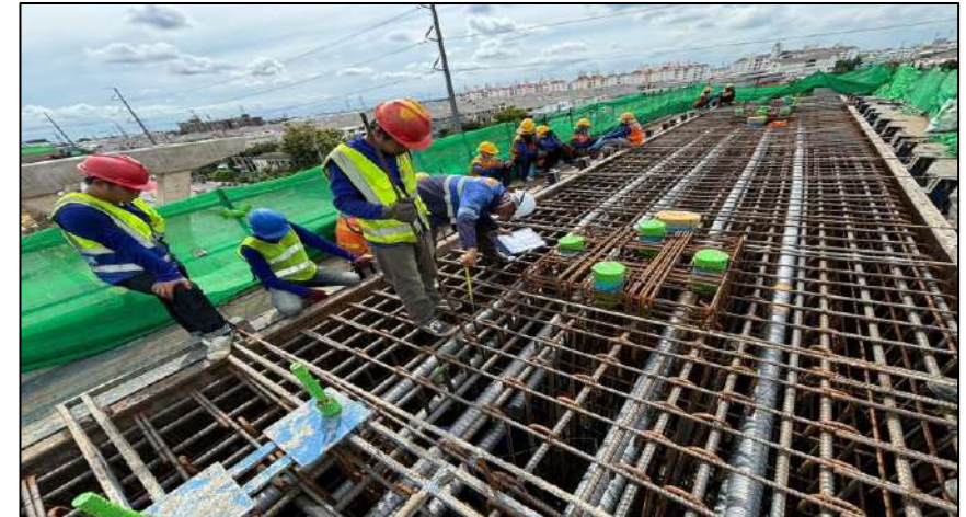
Install Steel Crossbeam Pier Type Y-1 MLP05-16C
