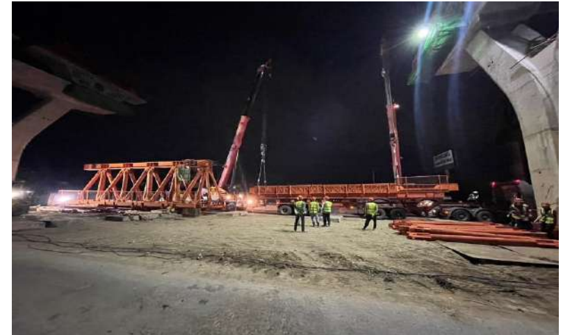
MLP01-31 to MLP01-32 Assembly Main truss (LG-5,6)
