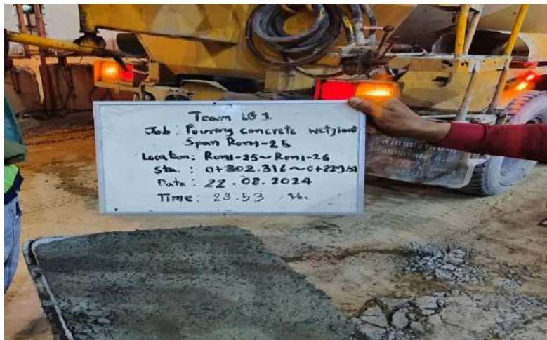
RON1-25 to RON1-26 Pouring concrete wet joint viaduct segment (LG1)
