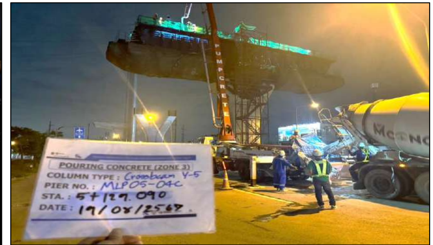
Pouring Concrete Crossbeam Pier Type Y-5 MLP05-04C Step 2
