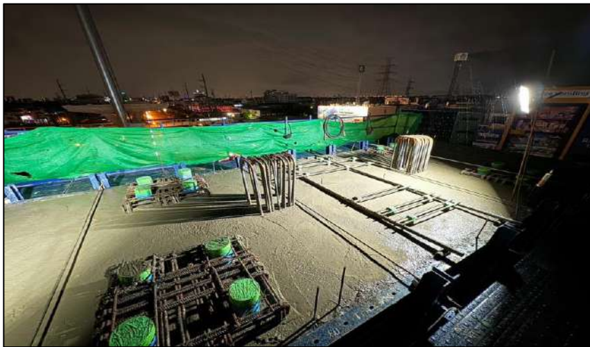
Pouring Concrete Crossbeam Pier Type Y-5 MLP05-04C Step 2
