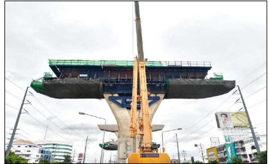
Install Steel Crossbeam Pier Type Y-1 MLP05-14C
