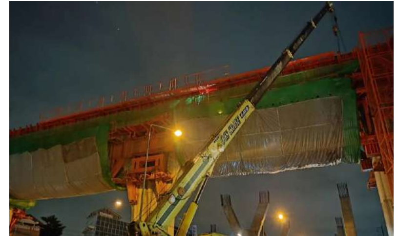
MLP01-24 งานติดตั้ง Formwork Side For Crossbeam Type IYI-4
