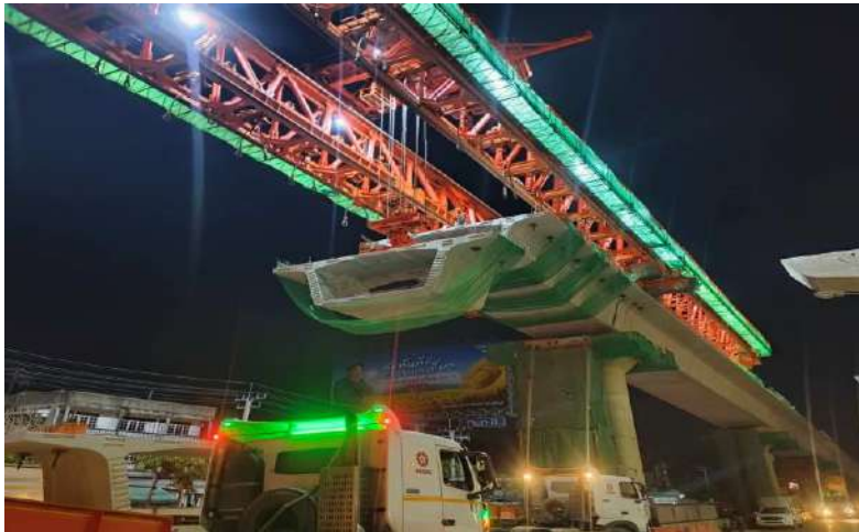
ROF1-03 to ROF1-04 Erection Viaduct Segment Span (LG2)
