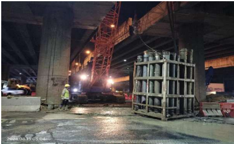
MLP03-09/2C Airlift Barrette Pile 2.80x0.80 m.
