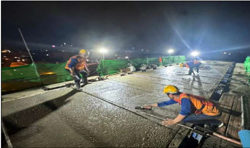
Pouring Concrete Crossbeam Pier Type Y-1 MLP05-13C
