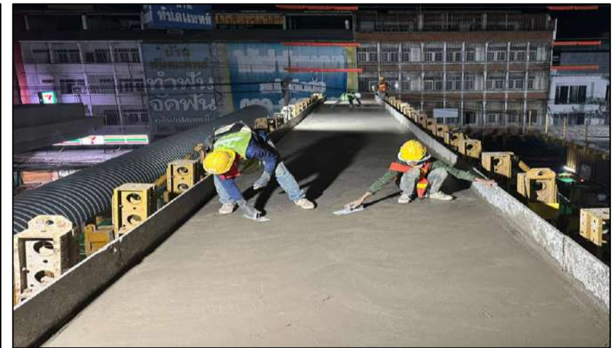
Pouring Concrete Crossheads Pier Type PTT-1 MLP04-18 Step 2
