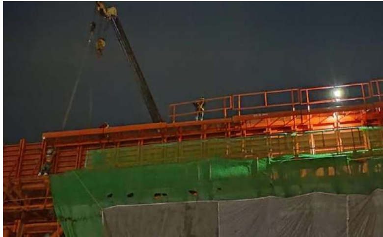
MLP01-24 งานติดตั้ง Formwork Side For Crossbeam Type IYI-4
