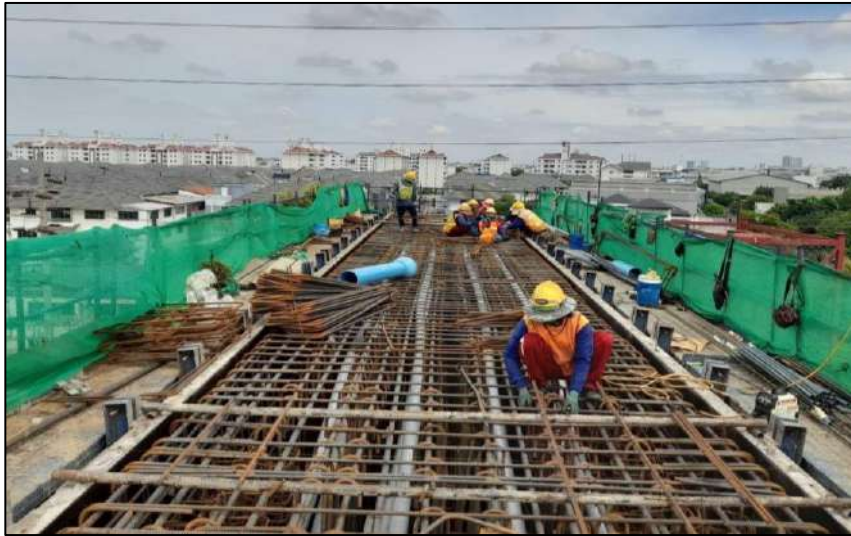
Install Steel Crossbeam Pier Type Y-1 MLP05-14C
