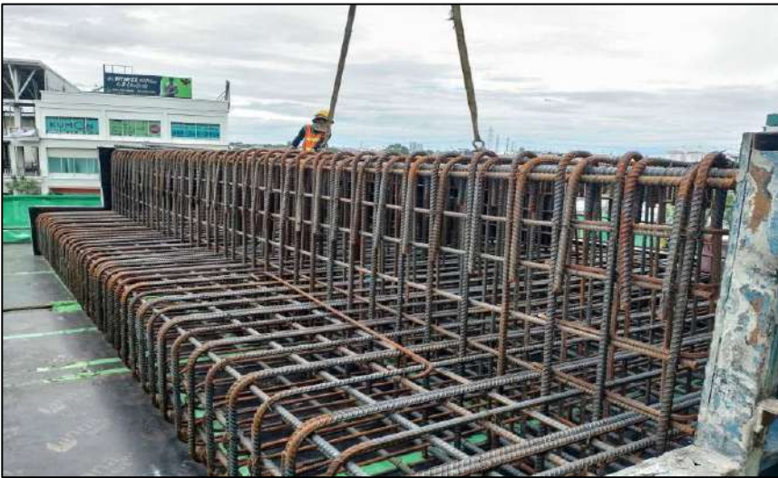
Install Steel Crossheads Pier Type P-1 ROF2-21
