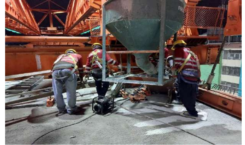
ROF2-06 Pouring concrete wet joint segment span (LG-3)
