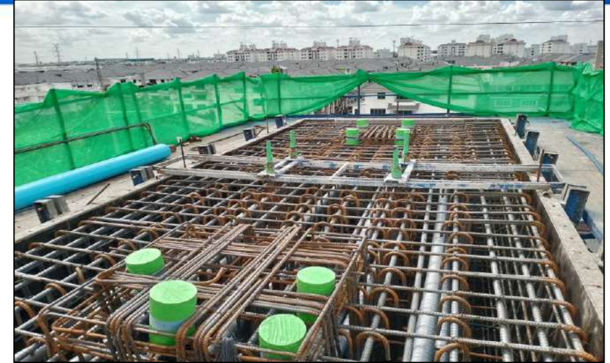
Install Steel Crossbeam Pier Type Y-1 MLP05-13C
