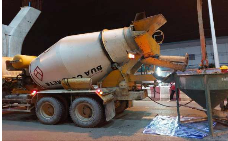
ROF2-06 Pouring concrete wet joint segment span (LG-3)
