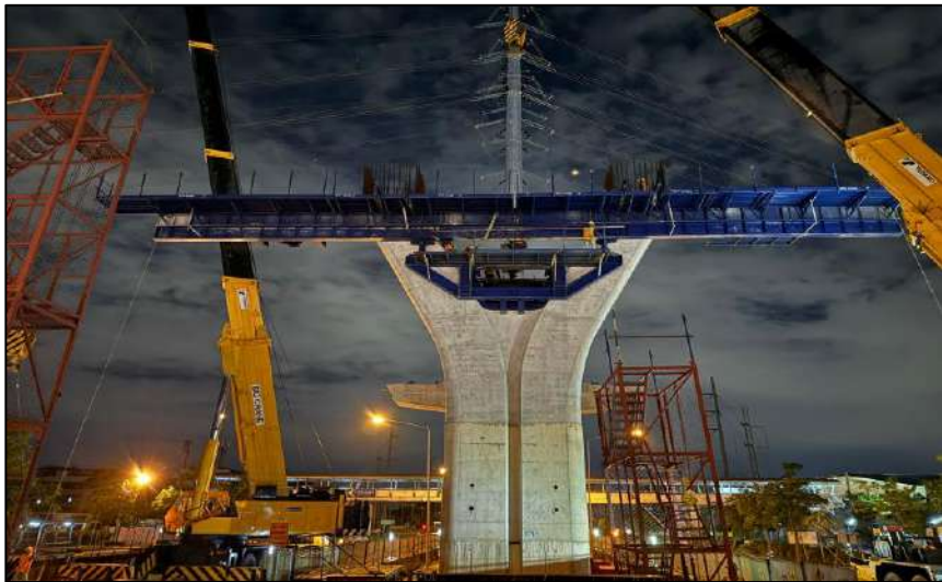
Install Support Formwork Crossbeam Pier Type Y-5 MLP05-05C
