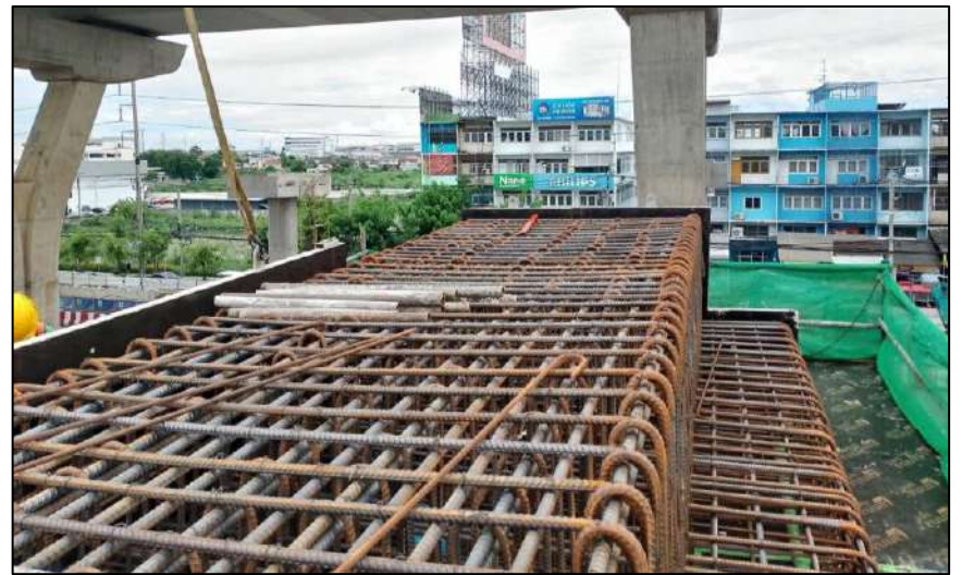
Install Steel Crossheads Pier Type P-1 ROF2-21
