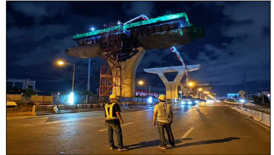
Pouring Concrete Crossbeam Pier Type Y-1 MLP05-13C
