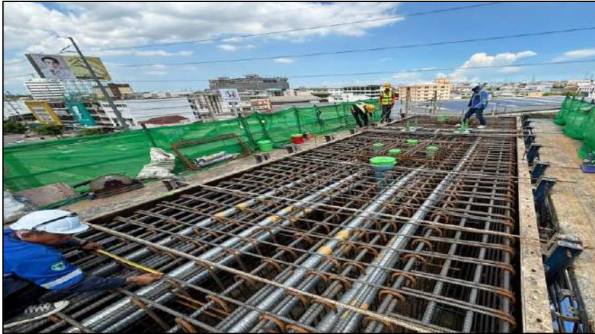
Install Steel Crossbeam Pier Type Y-1 MLP05-13C
