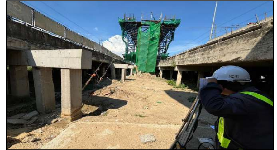
Install Steel Column Pier Type Y-5 Step Y MLP06-07C
