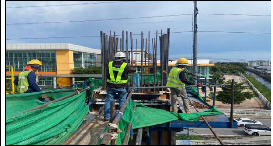
Install Steel Column Pier Type Y-5 Step Y MLP06-08C
