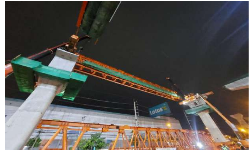
RON2-22 to RON2-23 Installation Main Truss (LG-4)
