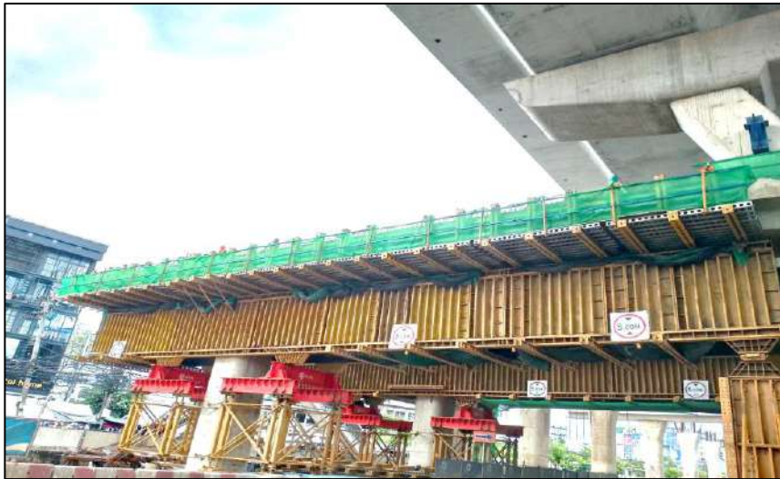
Install Steel Crossheads Pier Type YT-1 MLP04-17
