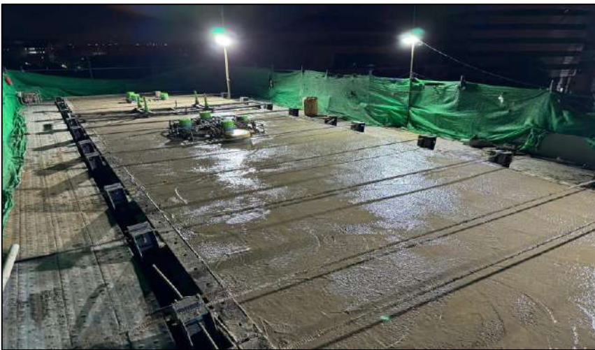
Pouring Concrete Crossbeam Pier Type Y-1 MLP05-16C
