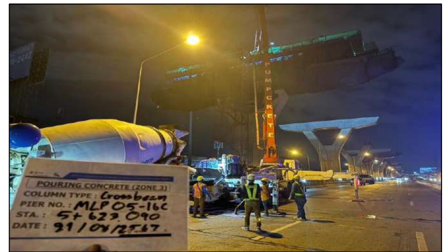
Pouring Concrete Crossbeam Pier Type Y-1 MLP05-16C
