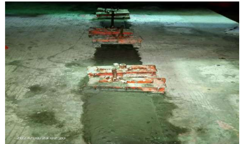
RON1-25 to RON1-26 Pouring concrete wet joint viaduct segment (LG1)
