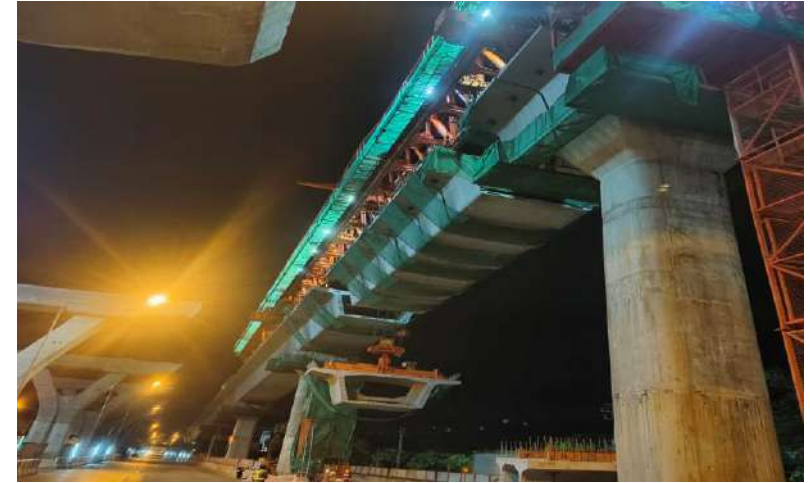
RON1-25 to RON1-26 Erection Viaduct Segment Span (LG1)
