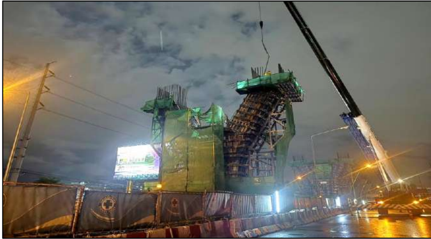
Install Steel Column Pier Type Y-5 Step Y MLP06-08C
