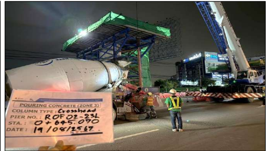
Pouring Concrete Crossheads Pier Type P-1 ROF2-23
