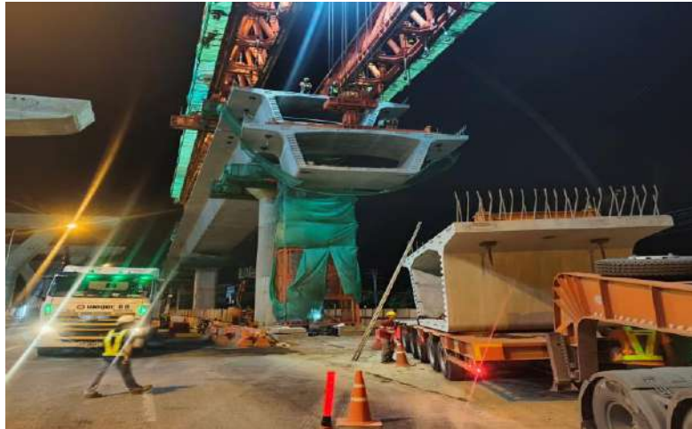
RON1-25 to RON1-26 Erection Viaduct Segment Span (LG1)
