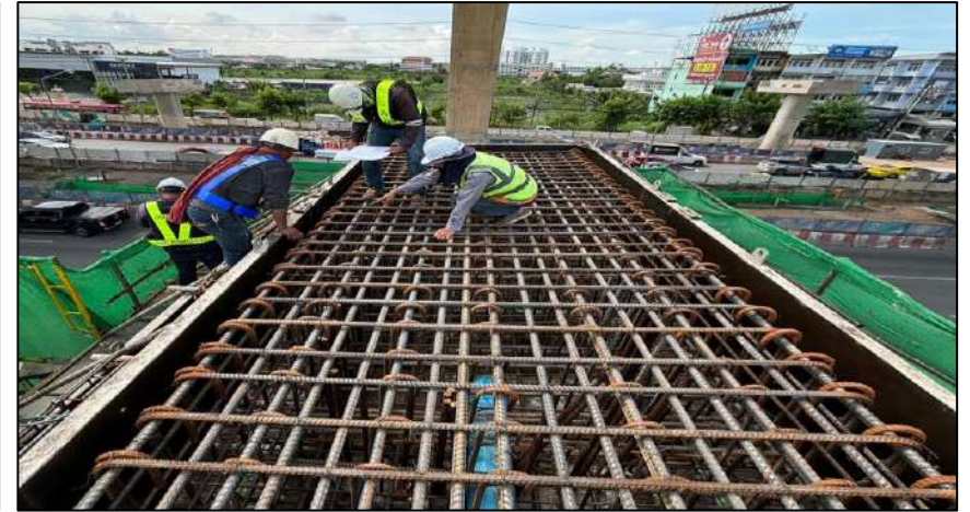
Install Steel Crossheads Pier Type P-1 ROF2-23
