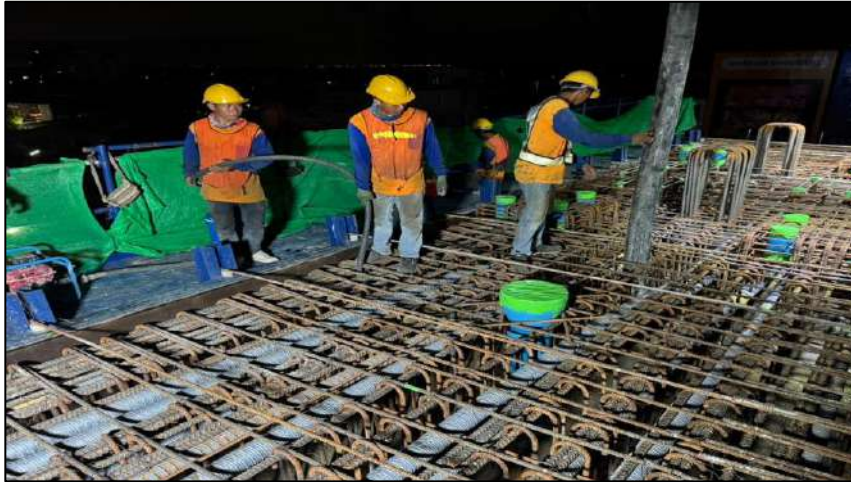
Pouring Concrete Crossbeam Pier Type Y-5 MLP05-04C Step 1
