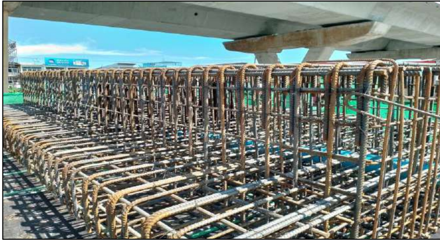
Install Steel Crossheads Pier Type P-1 ROF2-23
