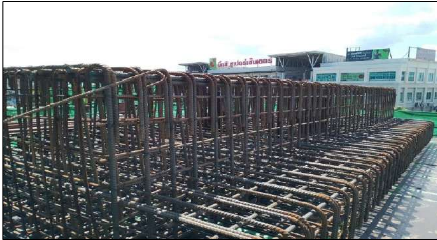
Install Steel Crossheads Pier Type P-1 ROF2-22
