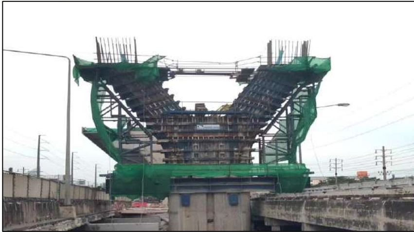
Install Steel Column Pier Type Y-5 Step Y MLP06-09C
