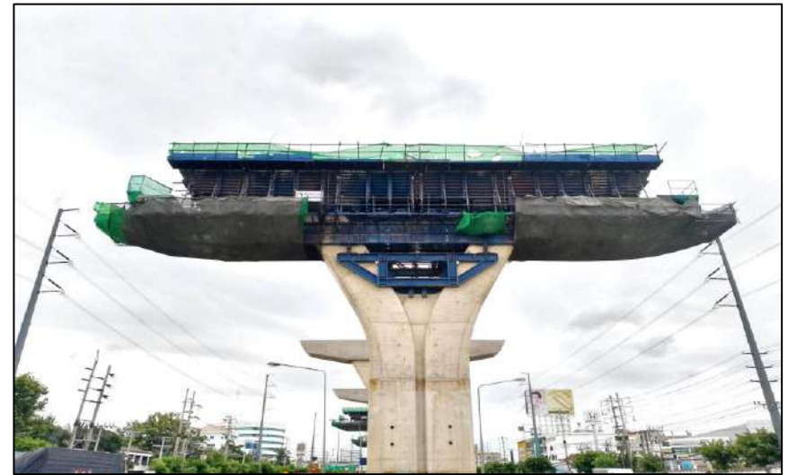
Install Steel Crossbeam Pier Type Y-1 MLP05-11C
