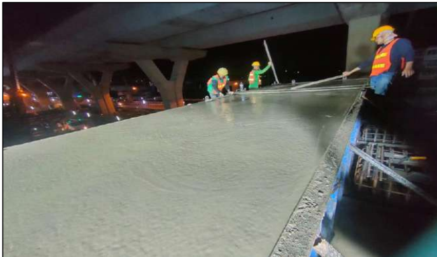
Pouring Concrete Crossheads Pier Type P-1 ROF2-22
