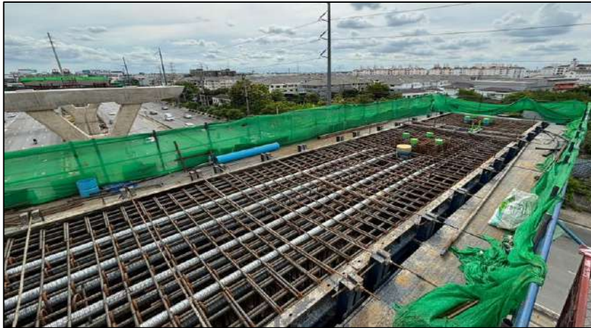
Install Steel Crossbeam Pier Type Y-1 MLP05-16C
