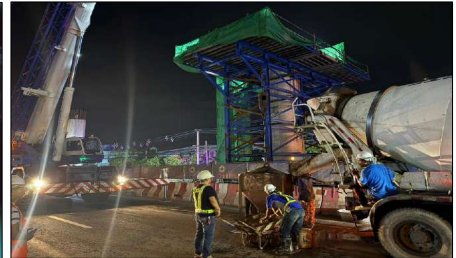
Pouring Concrete Crossheads Pier Type P-1 ROF2-22
