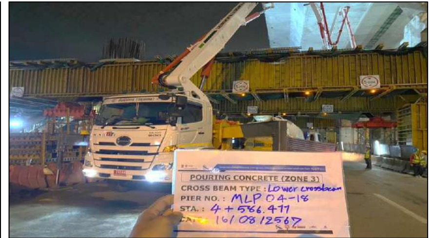
Pouring Concrete Crossheads Pier Type PTT-1 MLP04-18 Step 1
