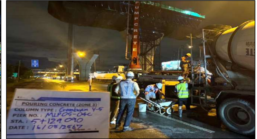
Pouring Concrete Crossbeam Pier Type Y-5 MLP05-04C Step 1
