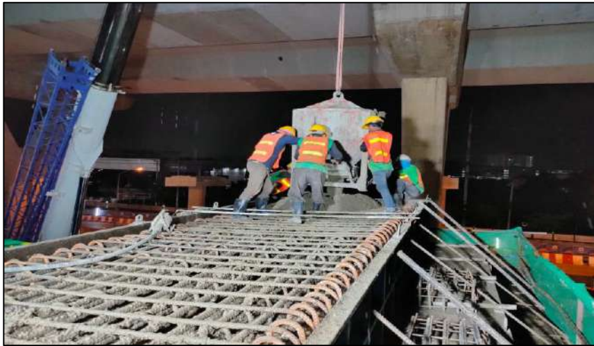
Pouring Concrete Crossheads Pier Type P-1 ROF2-23
