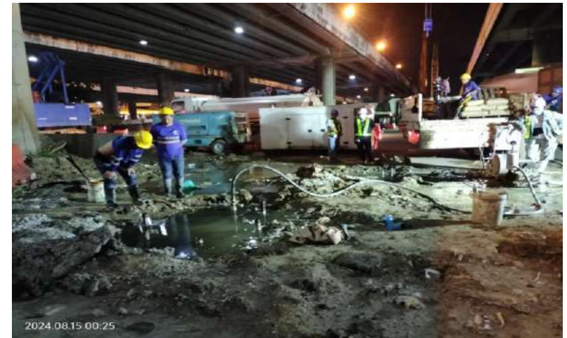
MLP03-09/2C Airlift Barrette Pile 2.80x0.80 m.
