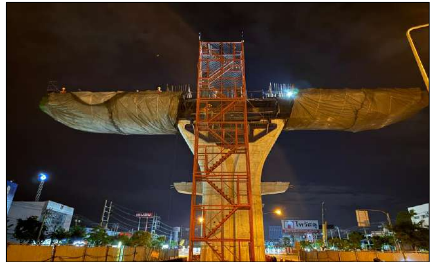
Install Support Formwork Crossbeam Pier Type Y-5 MLP05-05C
