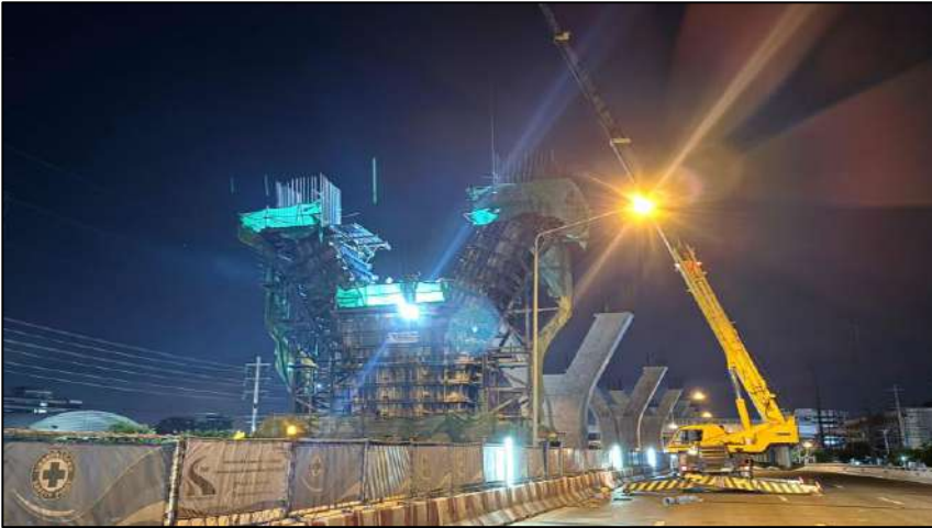
Install Steel Column Pier Type Y-5 Step Y MLP06-07C
