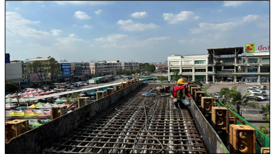
Install Steel Crossheads Pier Type YT-1 MLP04-22
