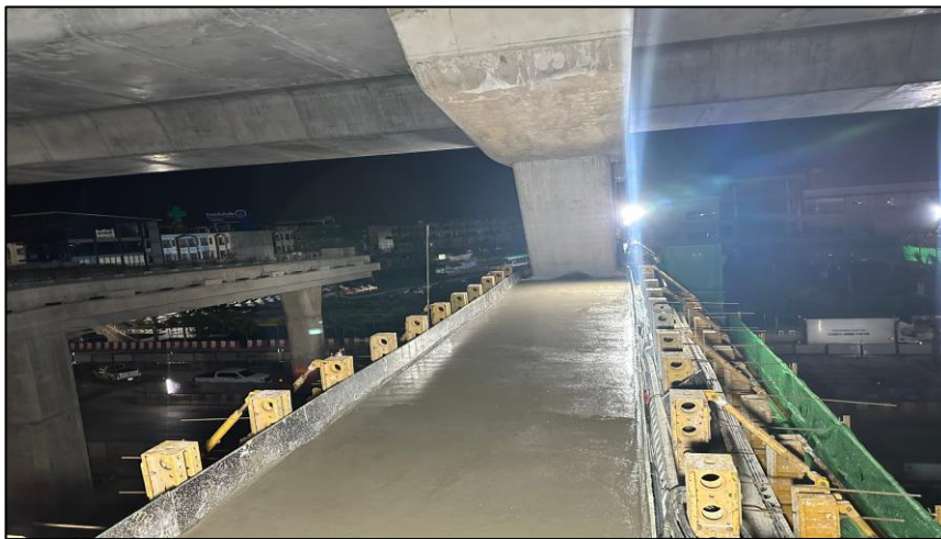
Pouring Concrete Crossheads Pier Type YT-1 MLP04-22 Step 2
