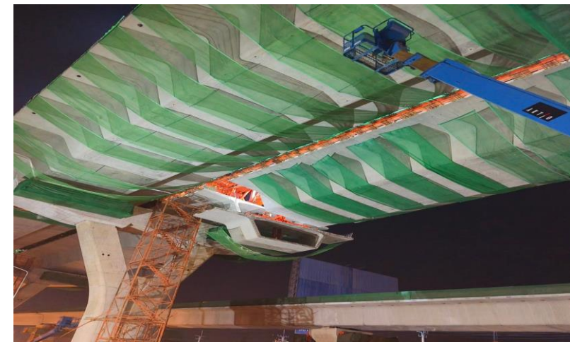
MLP01-16 to MLP01-17 Erection segment (LG1, 2)
