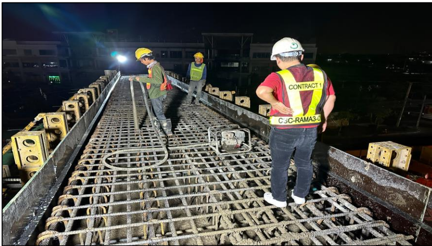
Pouring Concrete Crossheads Pier Type YT-2 MLP04-24 Step 2
