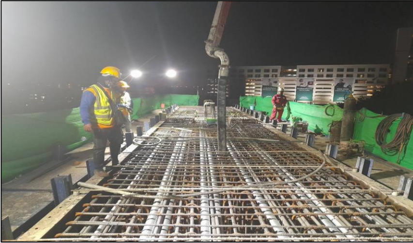
Pouring Concrete Crossbeam Pier Type Y-5 MLP06-10C Step 1
