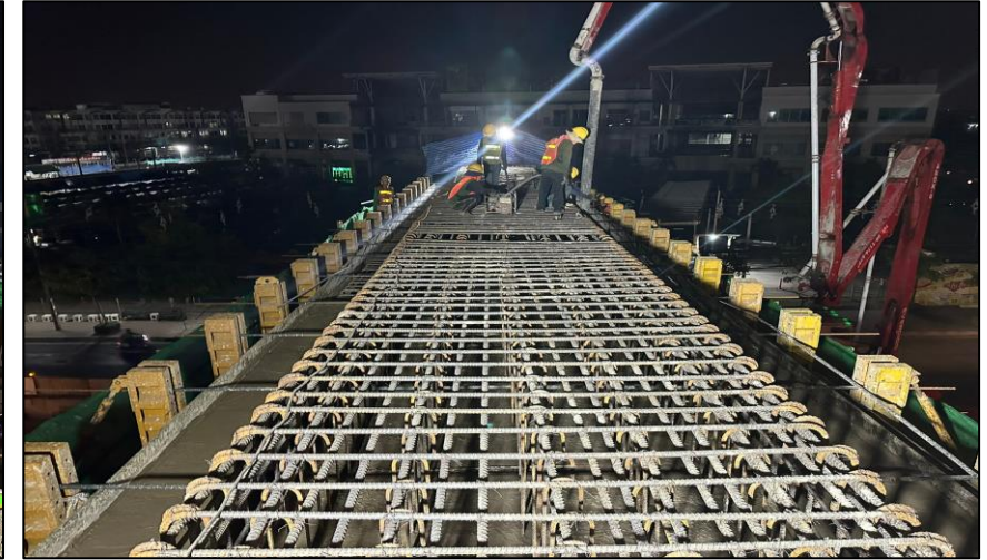
Pouring Concrete Crossheads Pier Type YT-2 MLP04-24 Step 1
