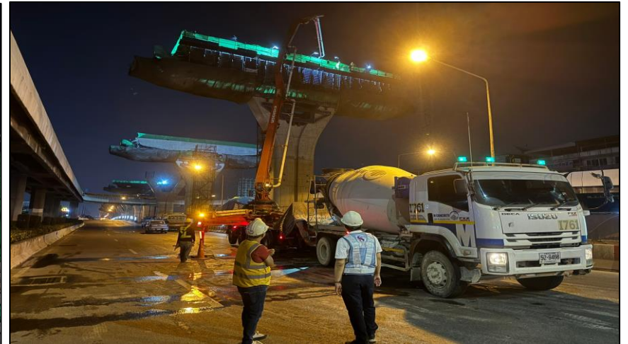
Pouring Concrete Crossbeam Pier Type Y-3 MLP05-26C
