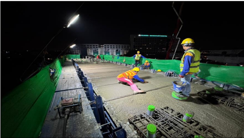
Pouring Concrete Crossbeam Pier Type Y-5 MLP06-10C Step 2
