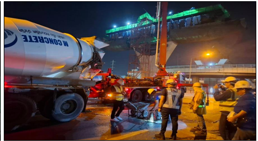
Pouring Concrete Crossbeam Pier Type Y-1 MLP06-04C
