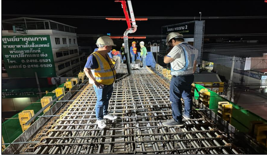
Pouring Concrete Crossheads Pier Type PTT-2 MLP04-23 Step 1
