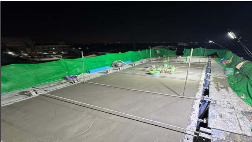
Pouring Concrete Crossbeam Pier Type Y-3 MLP05-26C
