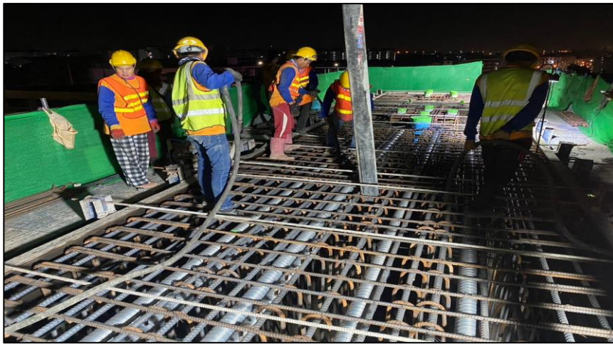
Pouring Concrete Crossbeam Pier Type Y-1 MLP06-02C
