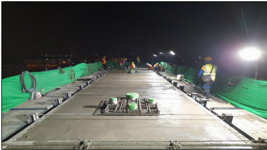
Pouring Concrete Crossbeam Pier Type Y-1 MLP06-04C
