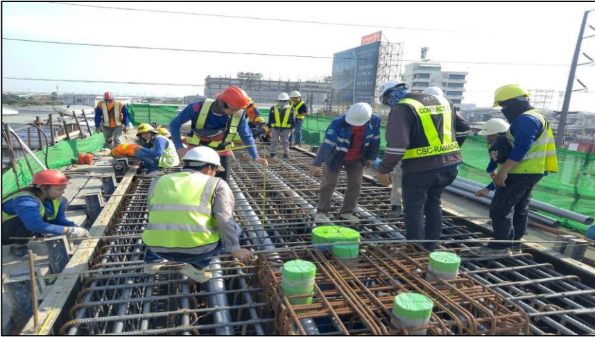
Install Steel Crossheads Pier Type Y-3 MLP05-26C
