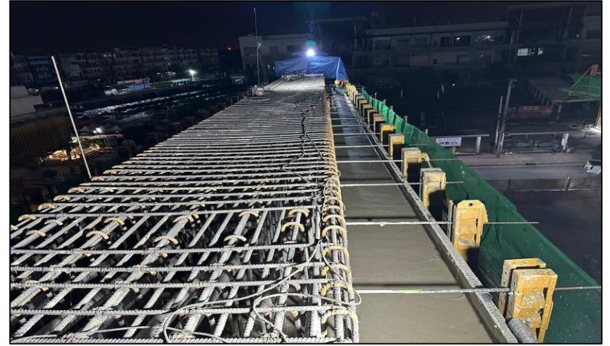
Pouring Concrete Crossheads Pier Type PTT-2 MLP04-23 Step 1
