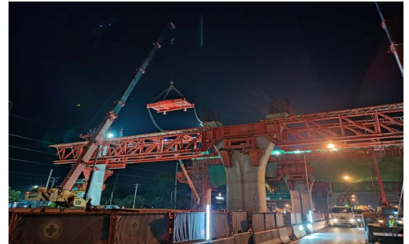
MLP02-15 งานติดตั้ง Formwork Crossbeam Type IYI-1
