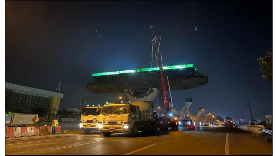
Pouring Concrete Crossbeam Pier Type Y-5 MLP06-10C Step 1
