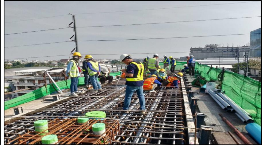
Install Steel Crossheads Pier Type Y-3 MLP05-26C
