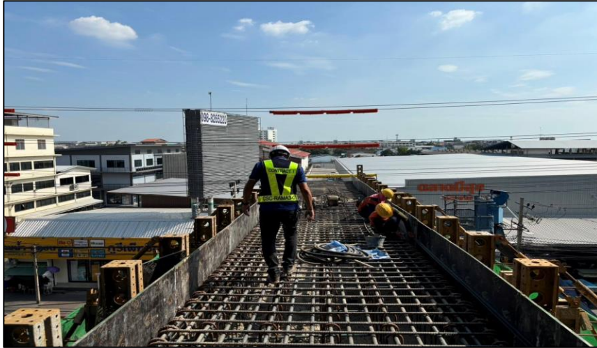
Install Steel Crossheads Pier Type YT-1 MLP04-22
