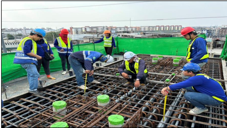
Install Steel Crossbeam Pier Type Y-1 MLP06-02C
