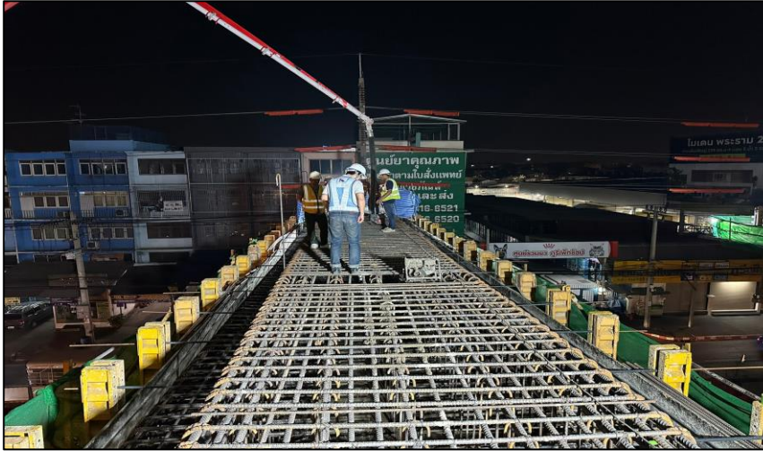
Pouring Concrete Crossheads Pier Type YT-2 MLP04-24 Step 1
