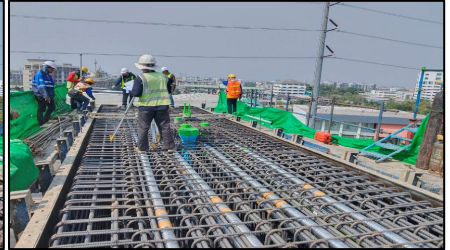
Install Steel Crossbeam Pier Type Y-1 MLP06-05C
