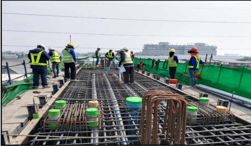
Install Steel Crossbeam Pier Type Y-1 MLP06-03C
