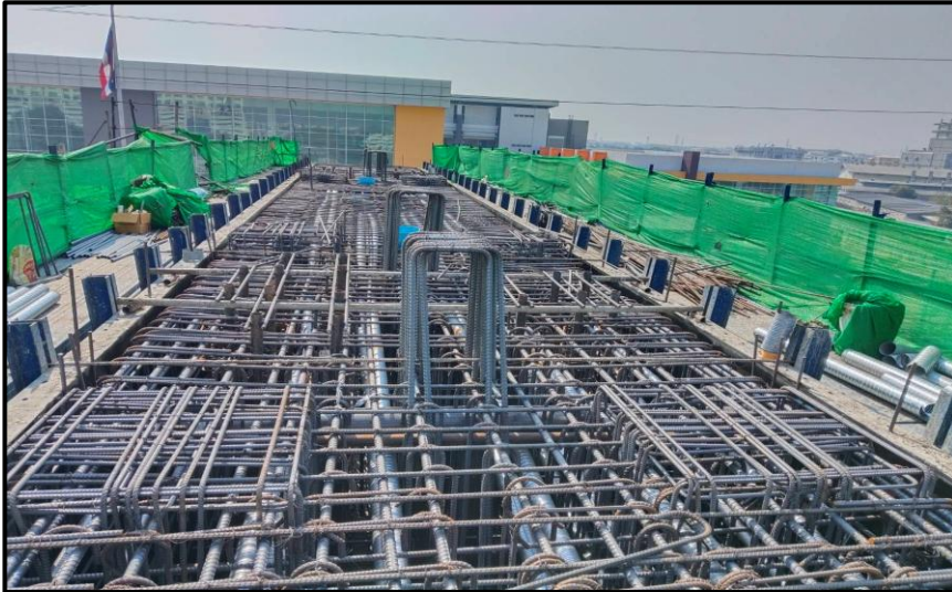
Install Steel Crossbeam Pier Type Y-5 MLP06-09C
