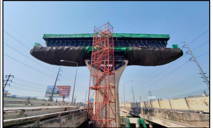
Install Steel Crossbeam Pier Type Y-5 MLP06-09C
