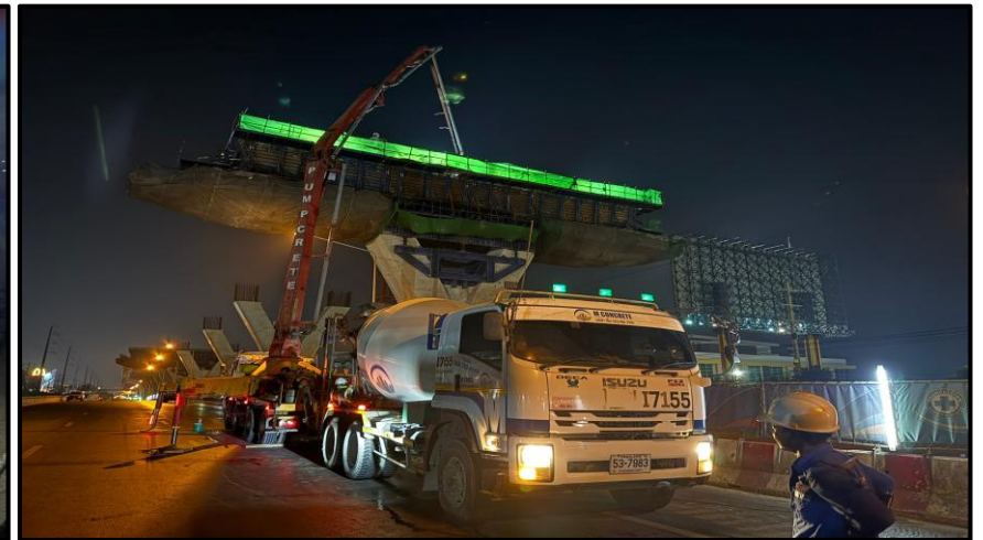
Pouring Concrete Crossbeam Pier Type Y-1 MLP06-05C
