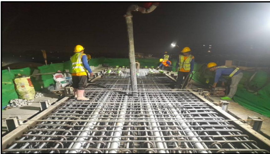
Pouring Concrete Crossbeam Pier Type Y-1 MLP06-03C
