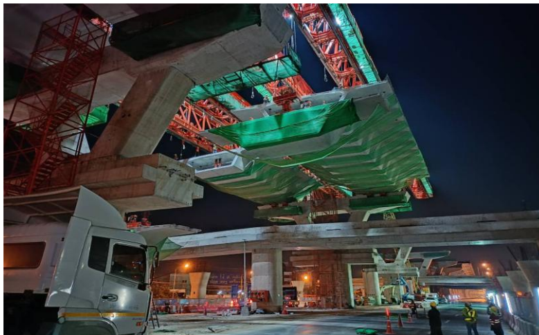
MLP01-08 to MLP01-09 Erection segment (LG1, 2)
