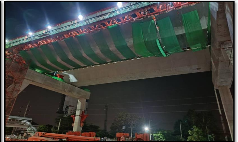
MLP02-16 to MLP02-17 Erection segment (LG7,8)
