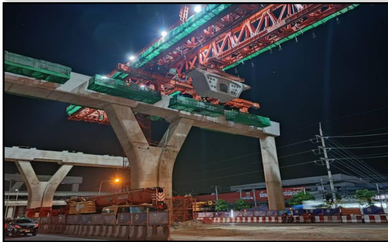
MLP01-24 to MLP01-25 Install Pier Segment (LG 2)
