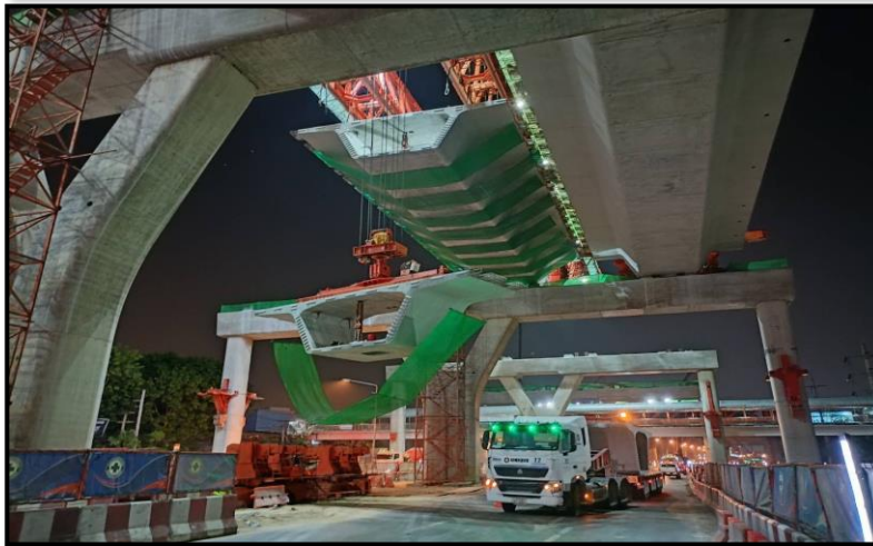
MLP02-16 to MLP02-17 Erection segment (LG7,8)
