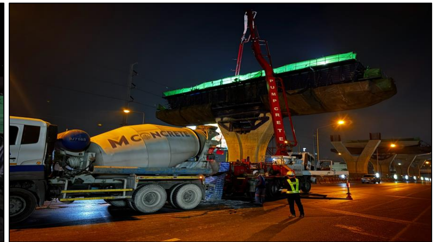
Pouring Concrete Crossbeam Pier Type Y-5 MLP06-08C Step 2
