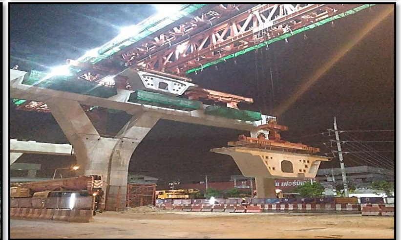
MLP01-24 to MLP01-25 Install Pier Segment (LG 2)
