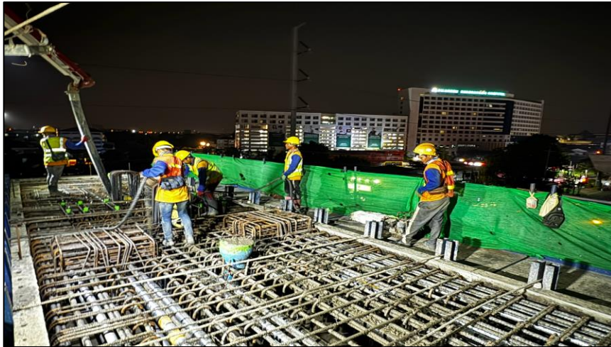
Pouring Concrete Crossbeam Pier Type Y-5 MLP06-08C Step 1
