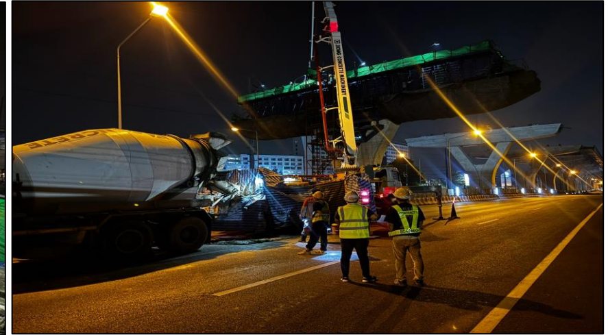
Pouring Concrete Crossbeam Pier Type Y-5 MLP06-08C Step 1
