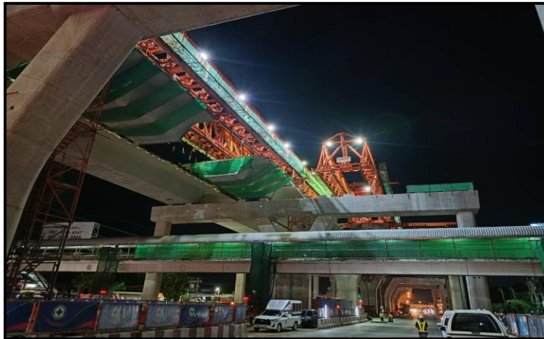
MLP02-18 to MLP02-19 Erection segment (LG8)
