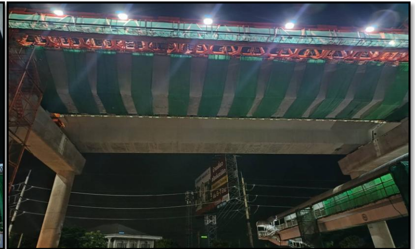
MLP02-18 to MLP02-19 Erection segment (LG8)
