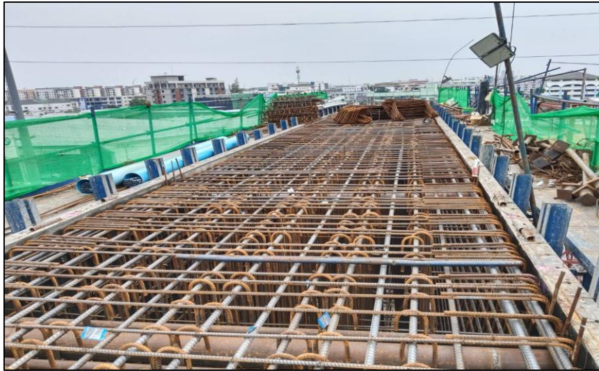
Install Steel Crossbeam Pier Type Y-5 MLP06-07C
