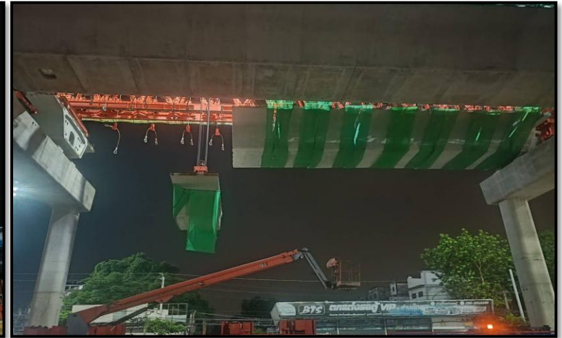
MLP02-16 to MLP02-17 Erection segment (LG7)
