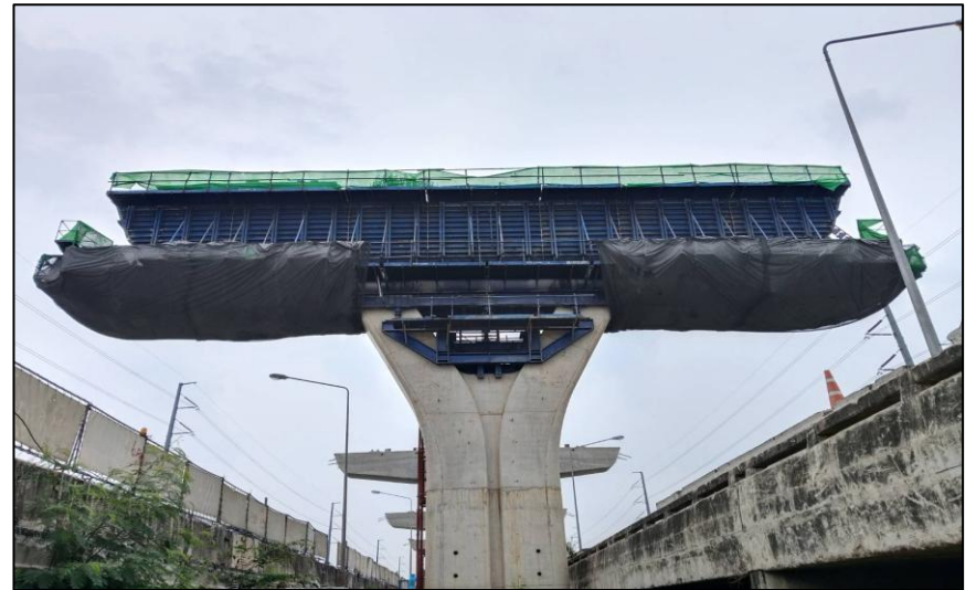
Install Steel Crossbeam Pier Type Y-5 MLP06-07C
