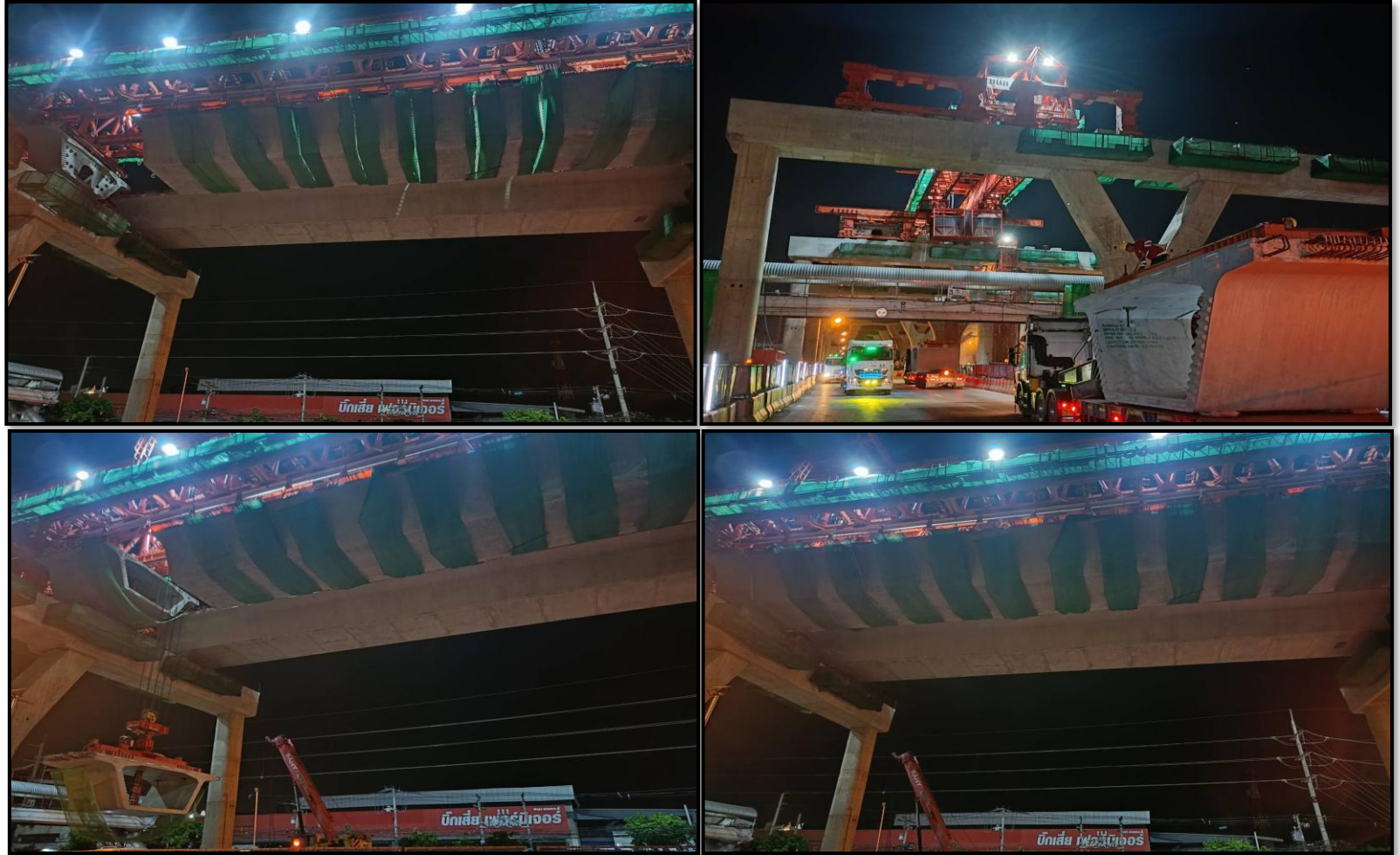
MLP01-25 to MLP01-26 Erection segment (LG2)
