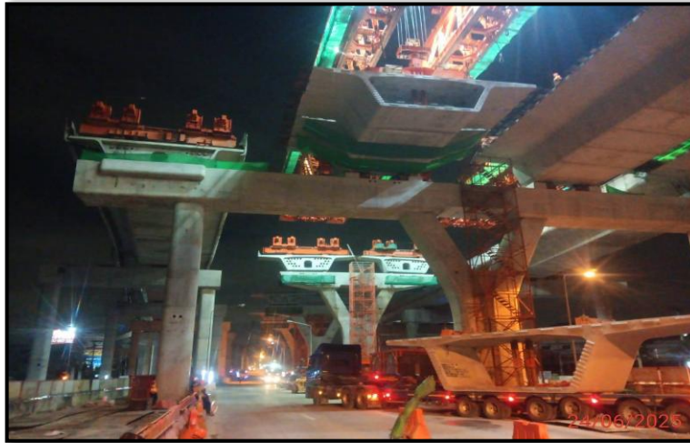
MLP02-20 to MLP02-21 Erection segment (LG7)
