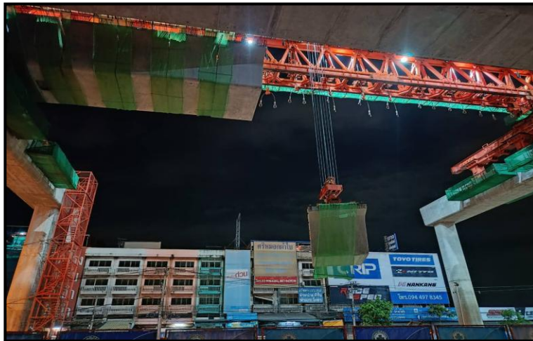
MLP01-27 to MLP01-28 Erection segment (LG1)
