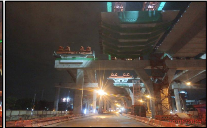
MLP02-20 to MLP02-21 Erection segment (LG7)
