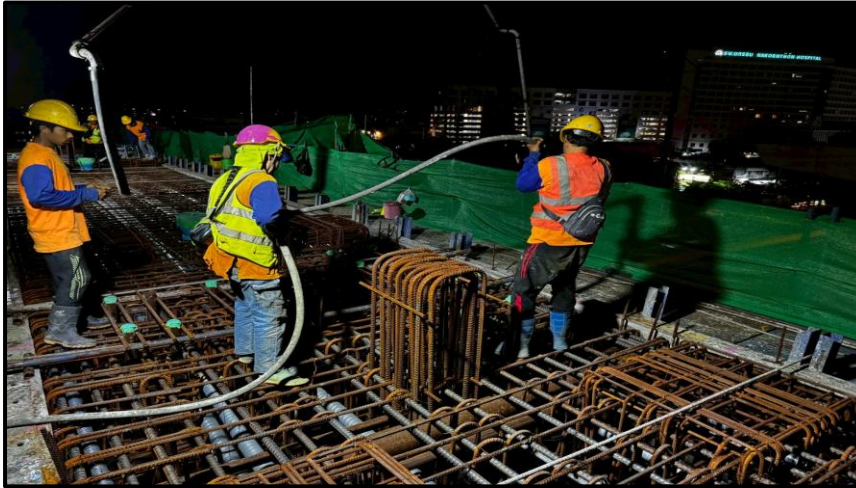
Pouring Concrete Crossbeam Pier Type Y-5 MLP06-07C Step 1
