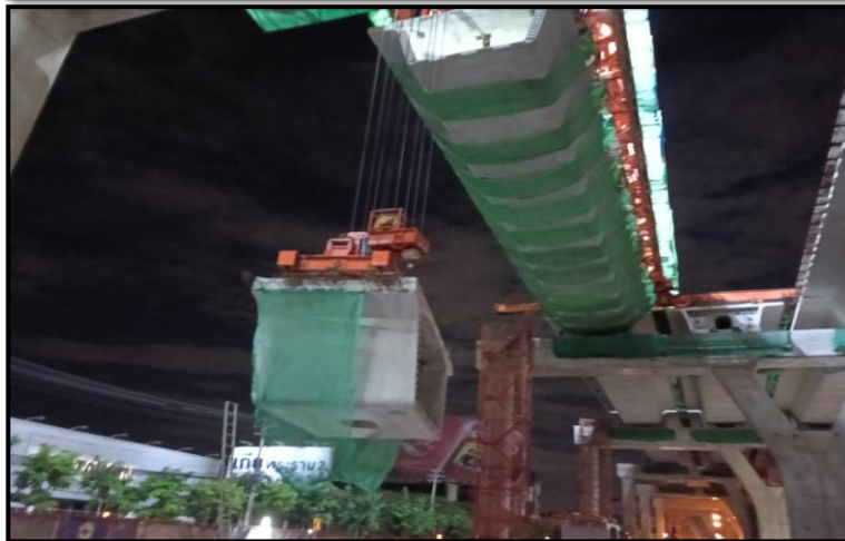
MLP03-28 to MLP04-01 Erection Segment (LG3)
