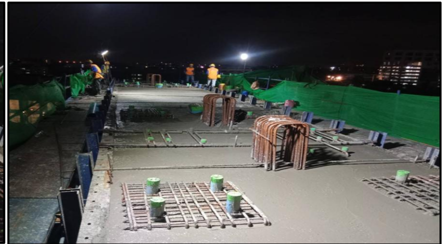
Pouring Concrete Crossbeam Pier Type Y-5 MLP06-07C Step 1
