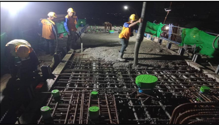
Pouring Concrete Crossbeam Pier Type Y-5 MLP06-07C Step 1
