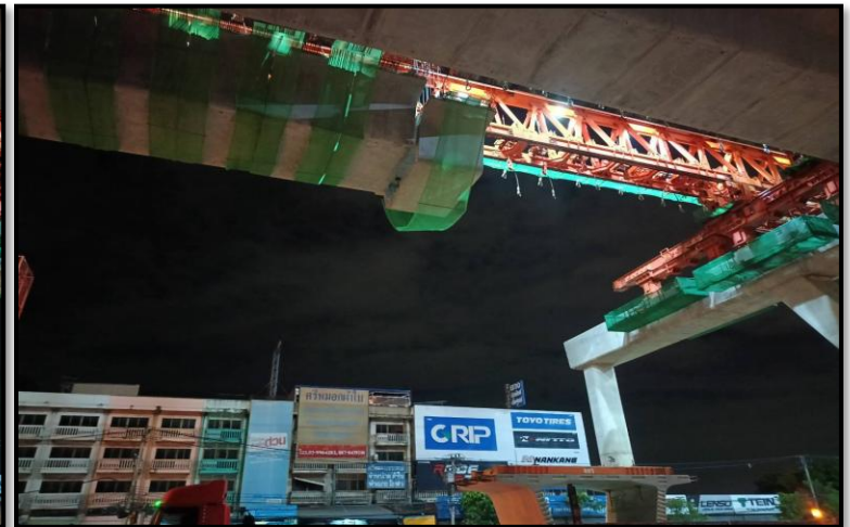
MLP01-27 to MLP01-28 Erection segment (LG1)
