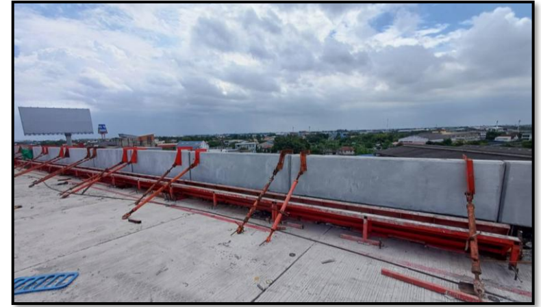
Install Side Formwork Precast Edge Parapet MLP02-05 to MLP02-06
