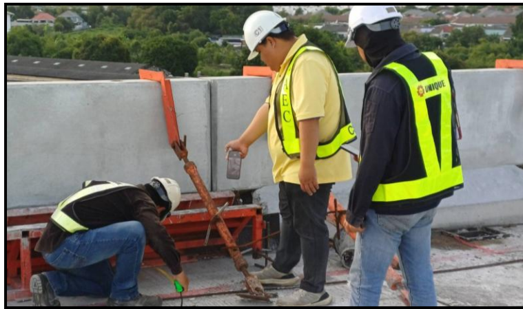
Final Inspection Precast Edge Parapet MLP01-27 to MLP01-28
