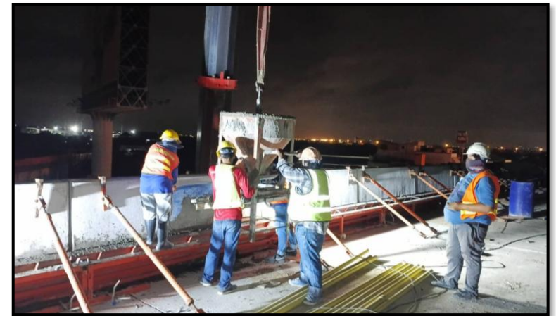
Infill Concrete Precast Edge Parapet MLP01-32 to MLP02-01
