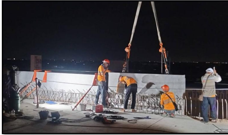
Install Precast Edge MLP01-27 to MLP01-28
