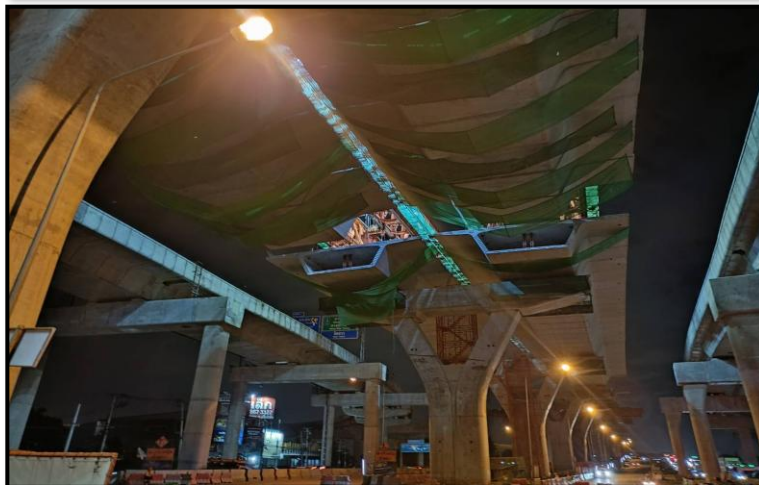
MLP02-22 to MLP02-23 Erection segment (LG7,8)
