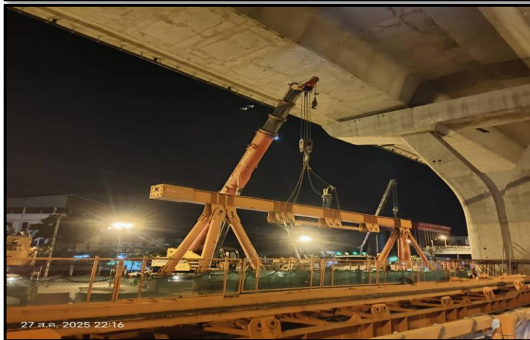
Dismantling the Launching Gantry Element (LG2)
