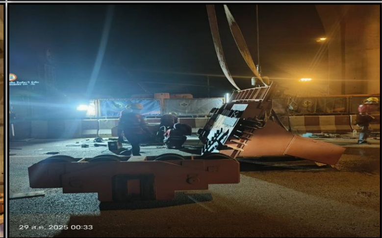
Dismantling the Launching Gantry Element (LG2)
