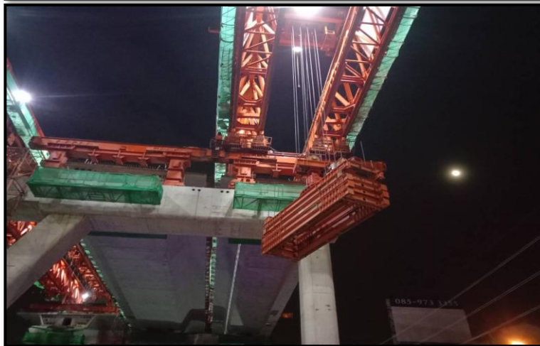
Prepare Launching Gantry to Next Span (LG3,4)
