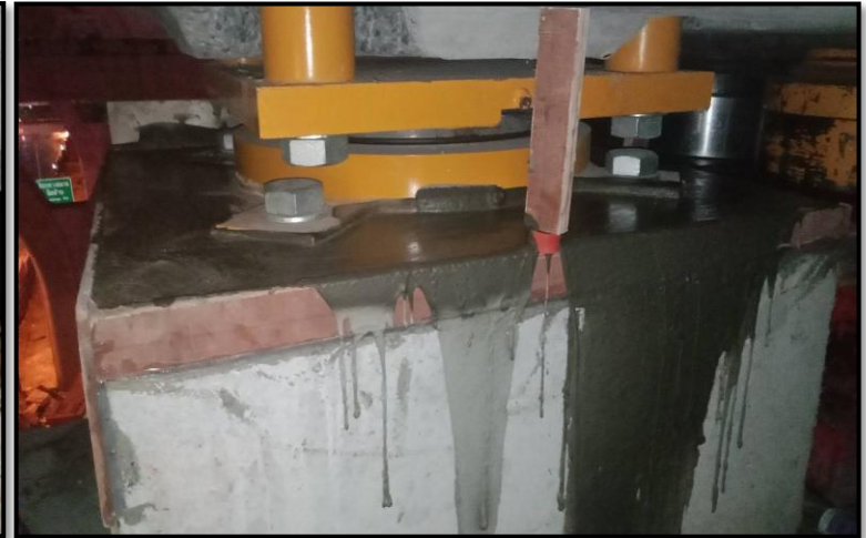
MLP02-21 to MLP02-22 Grouting Pot Bearing (LG7,8)
