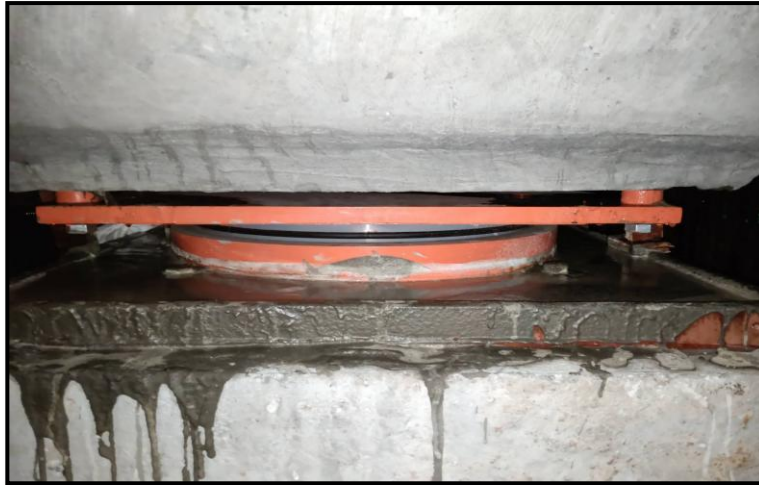
MLP02-21 to MLP02-22 Grouting Pot Bearing (LG7,8)
