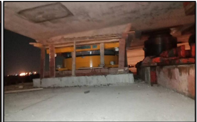
MLP02-21 to MLP02-22 Install Pot Bearing Formwork (LG7,8)
