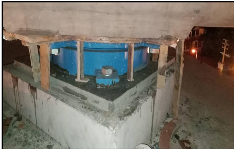
MLP02-21 to MLP02-22 Install Pot Bearing Formwork (LG7,8)
