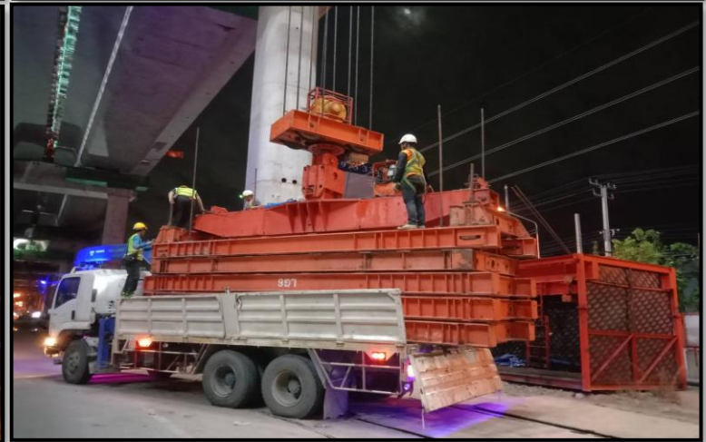
Prepare Launching Gantry to Next Span (LG3,4)
