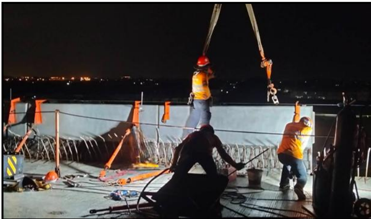
Install Precast Edge Parapet MLP01-29 to MLP01-30
