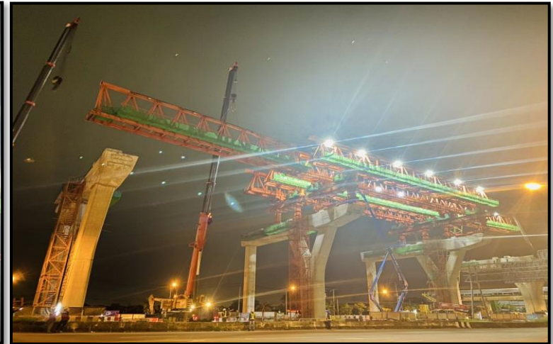
Erection Joint Element (LG1, 2)
