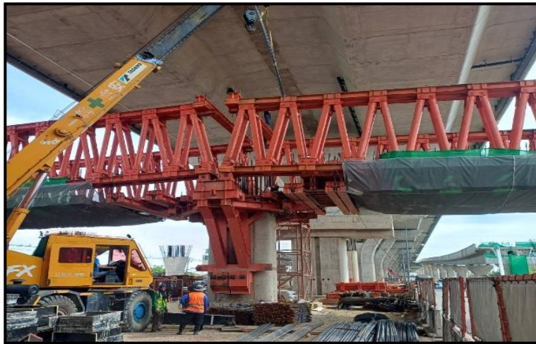
MLP01-12 Install Reinforcement Lower Crossbeam Type PTT-1
