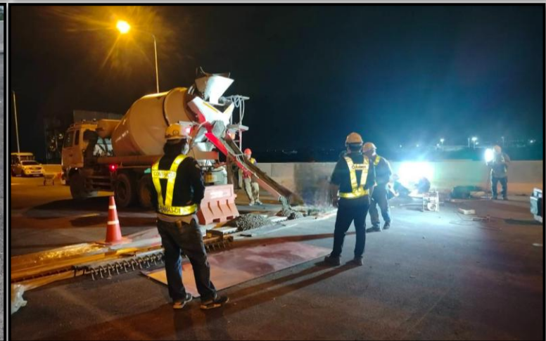
งาน Expansion Joint MLP01-26 to MLP02-21
