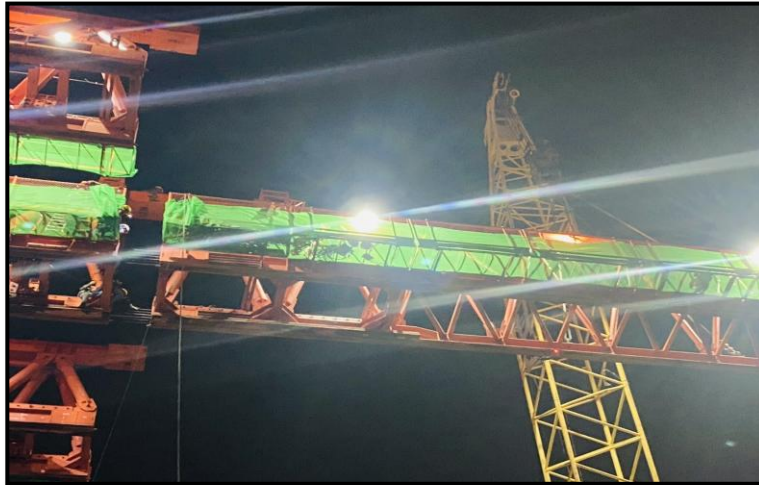
Erection Joint Element (LG1, 2)
