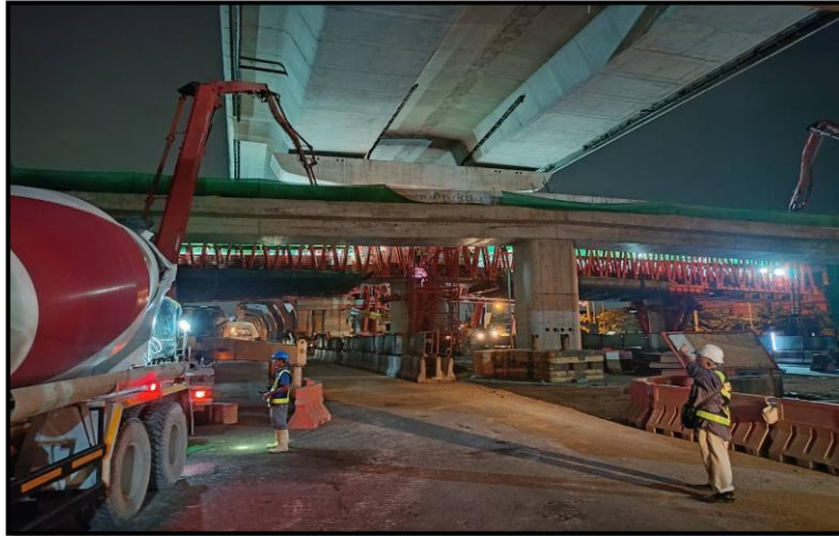
MLP01-11 Pouring Concrete Lower Crossbeam Type YT-1 Step 2
