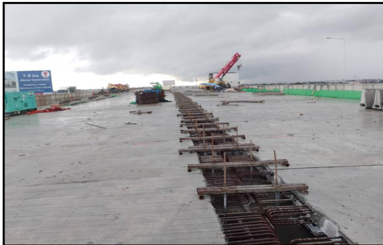
MLP02-21 to MLP02-22 Install Reinforcement Connecting Slab
