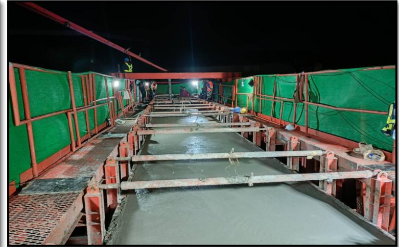
MLP01-11 Pouring Concrete Lower Crossbeam Type YT-1 Step 2
