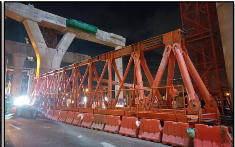
Assembly Bracing Element (LG1, 2)
