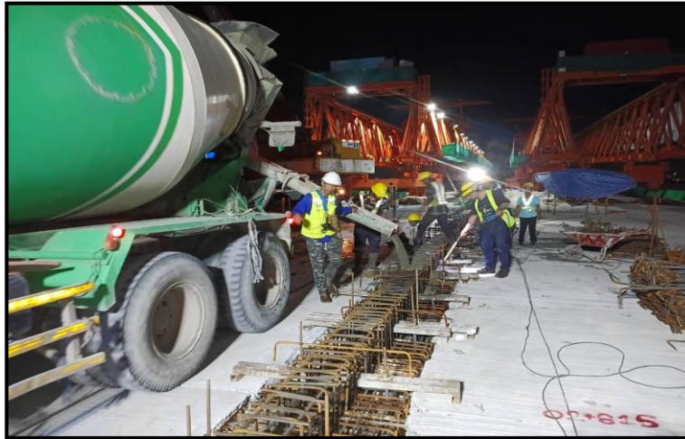
MLP02-20 to MLP02-21 Install Reinforcement Connecting Slab
