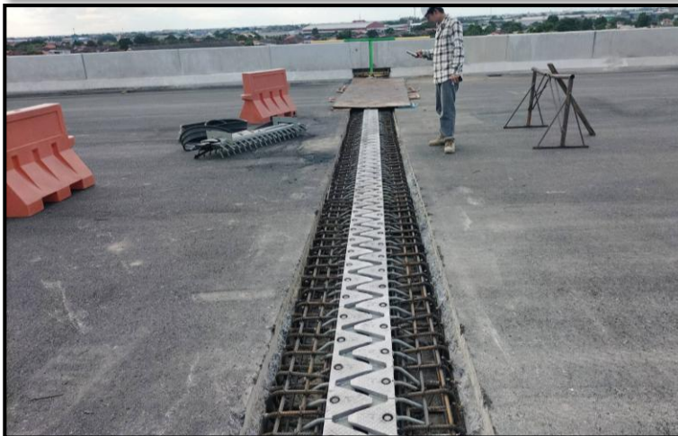
งาน Expansion Joint MLP01-26 to MLP02-21
