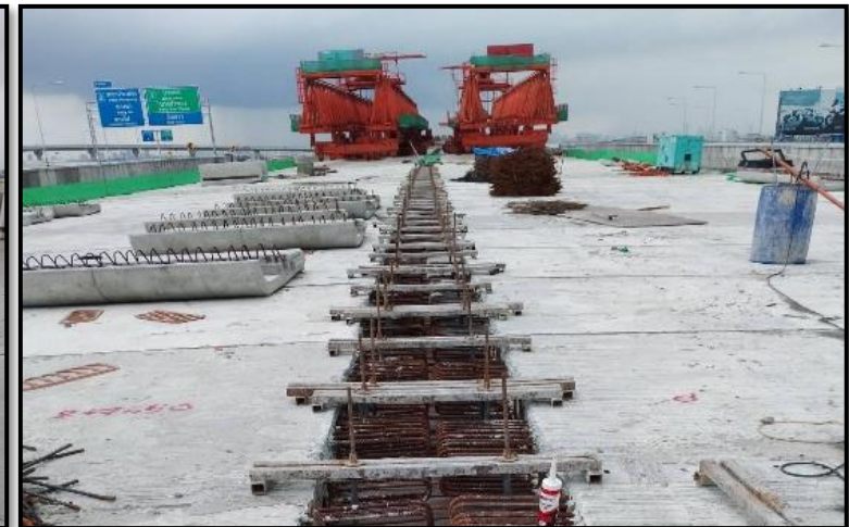
MLP02-21 to MLP02-22 Install Reinforcement Connecting Slab
