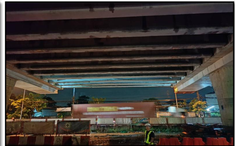
MLP01-07 to MLP01-08 Install Precast I-Girder
