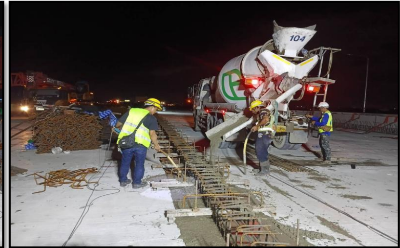
MLP02-20 to MLP02-21 Install Reinforcement Connecting Slab
