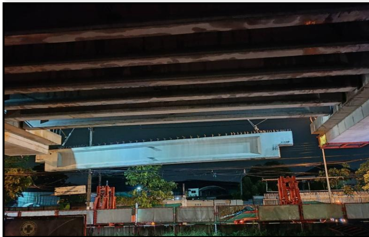
MLP01-07 to MLP01-08 Install Precast I-Girder
