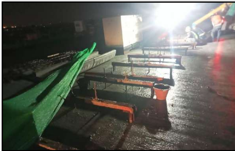
MLP03-23 to MLP03-24 Pouring Concrete Connecting Slab
