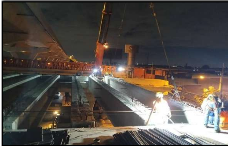
MLP01-09 to MLP01-10 Install Precast I-Girder
