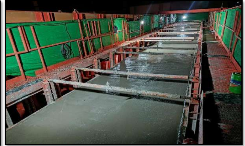
MLP01-12 Pouring Concrete Lower Crossbeam Type PTT-1
