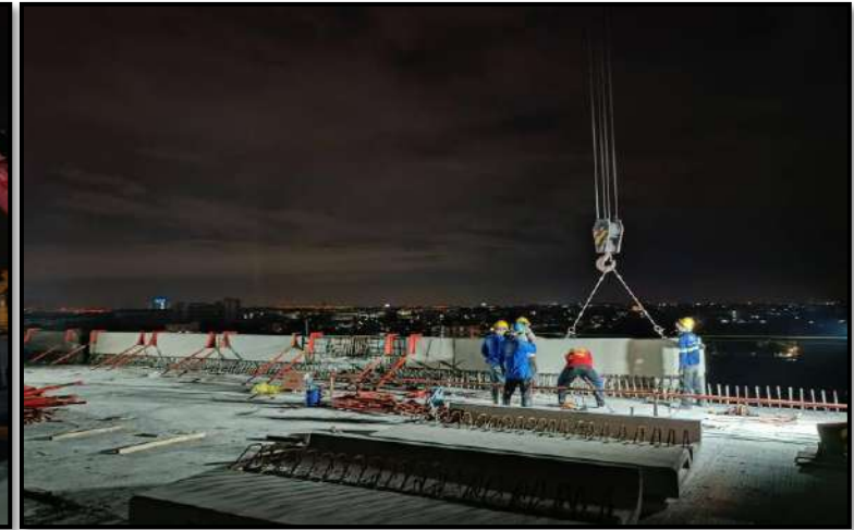
MLP03-26 to MLP3-27 Install Precast Edge Parapet
