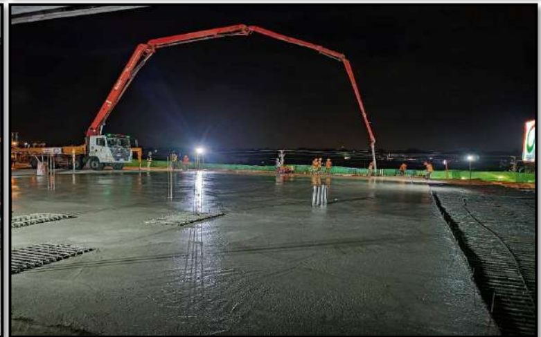
MLP01-07 to MLP01-08 Pouring Concrete Deck Slab
