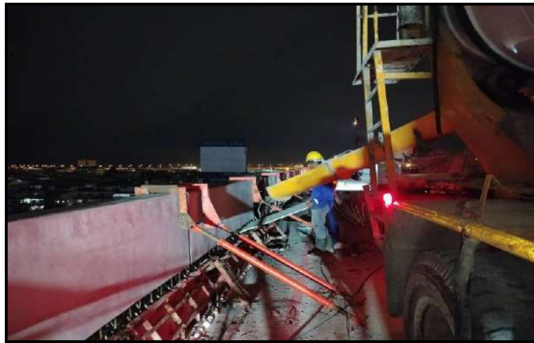
MLP03-28 to MLP04-01 Infill Concrete Precast Edge Parapet
