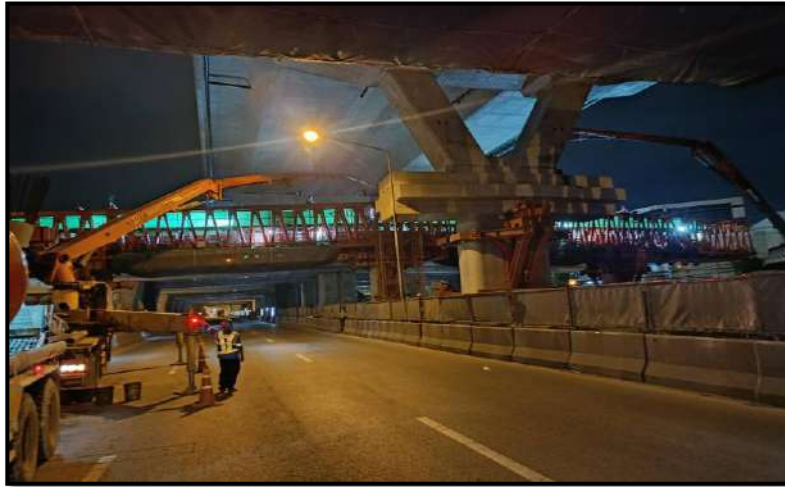
MLP01-12 Pouring Concrete Lower Crossbeam Type PTT-1
