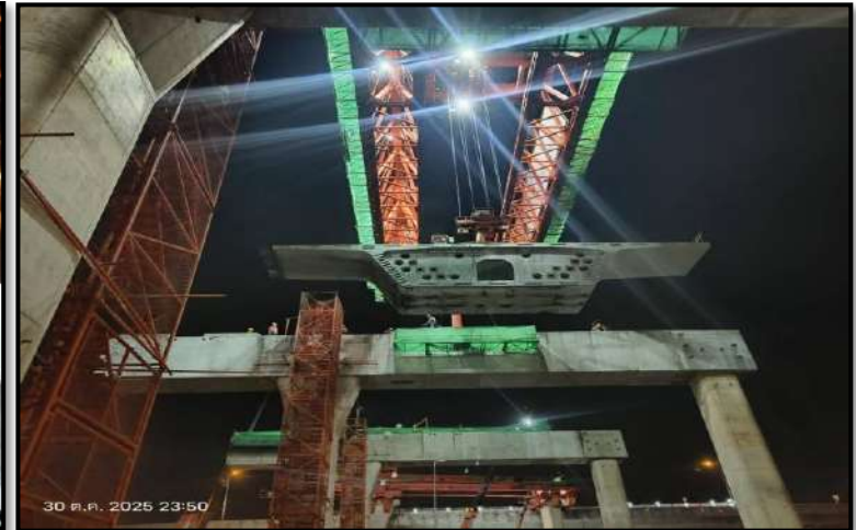
MLP03-15 Prepare Erection Segment Span (LG1)
