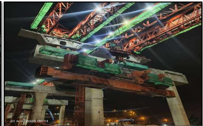
MLP03-17 to MLP03-18 Erection Segment Span (LG2)
