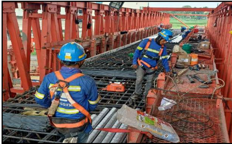
MLP01-14 Install Reinforcement Lower Crossbeam Type PTT-1
