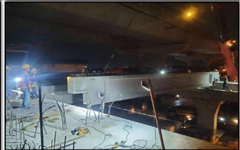
MLP01-09 to MLP01-10 Install Precast I-Girder
