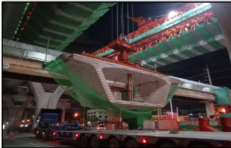
MLP03-21 to MLP03-22 Erection Segment Span (LG3,4)
