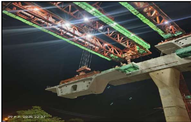
MLP03-17 to MLP03-18 Erection Segment Span (LG2)
