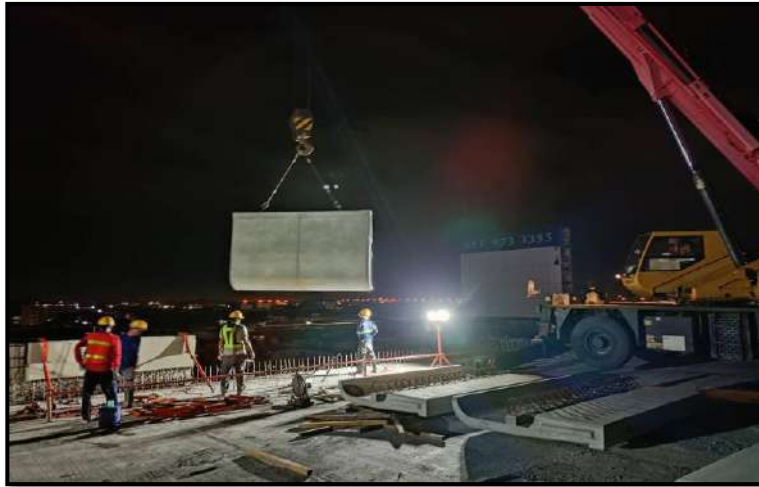
MLP03-26 to MLP3-27 Install Precast Edge Parapet
