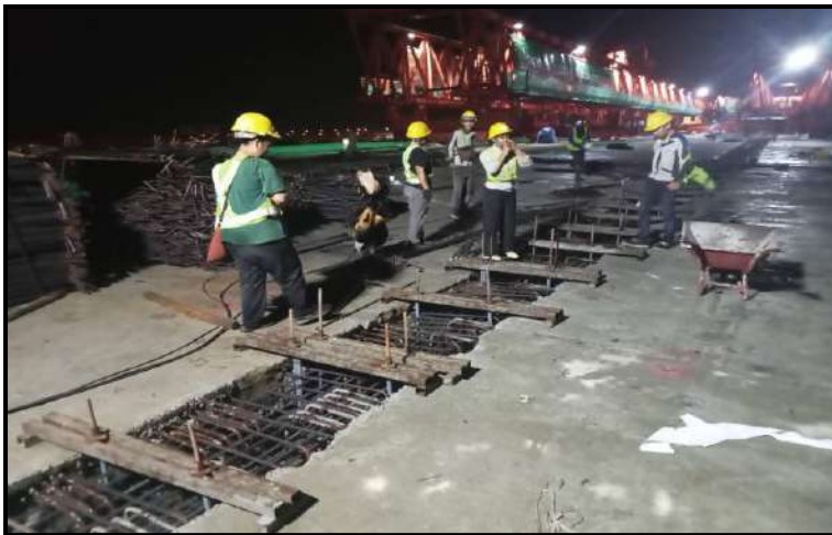
MLP03-23 to MLP03-24 Pouring Concrete Connecting Slab
