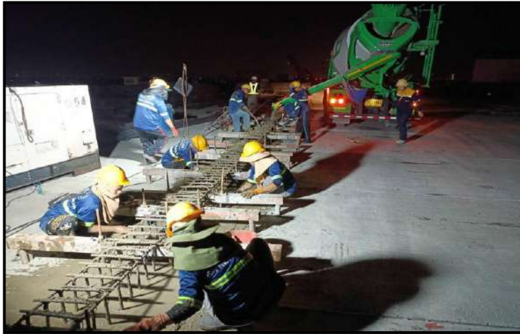
MLP03-22 to MLP03-23 Pouring Concrete Connecting Slab
