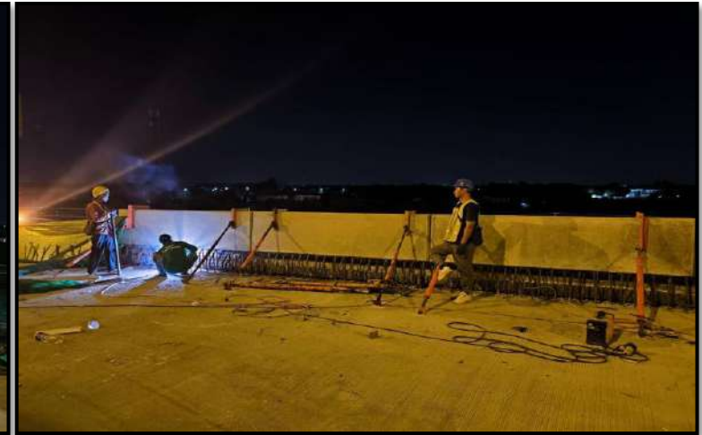
MLP01-03 to MLP01-04 Install Precast Edge Parapet
