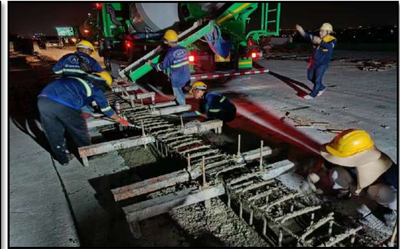
MLP03-22 to MLP03-23 Pouring Concrete Connecting Slab
