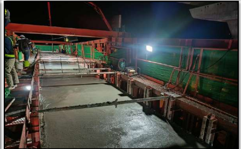
MLP01-14 Pouring Concrete Lower Crossbeam Type PTT-1
