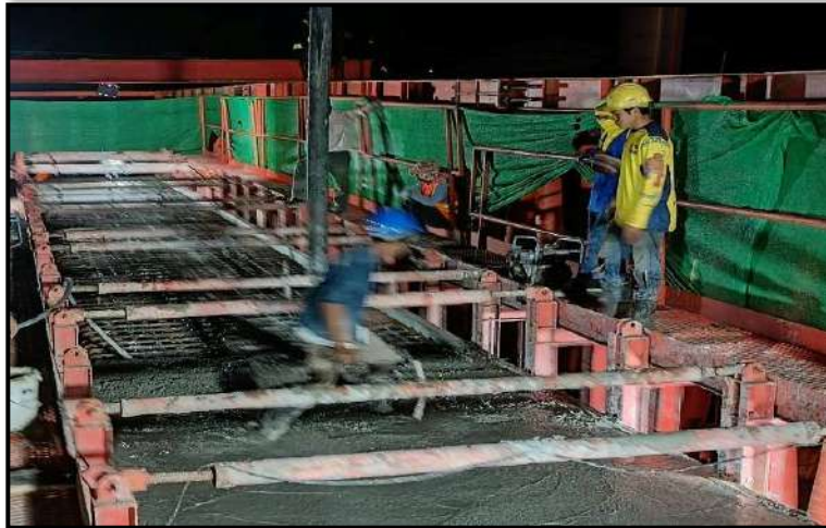
MLP01-14 Pouring Concrete Lower Crossbeam Type PTT-1
