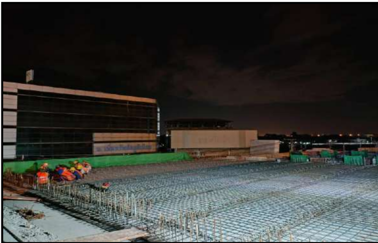
MLP01-09 to MLP01-10 Install Reinforcement Deck Slab
