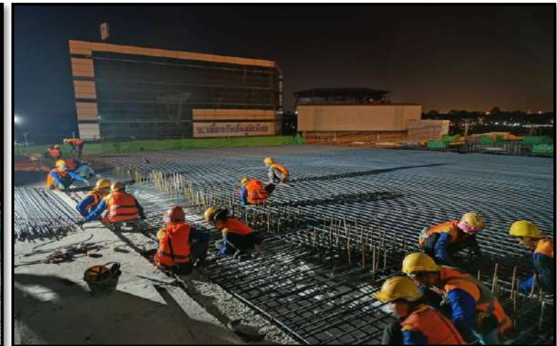
MLP01-09 to MLP01-10 Install Reinforcement Deck Slab
