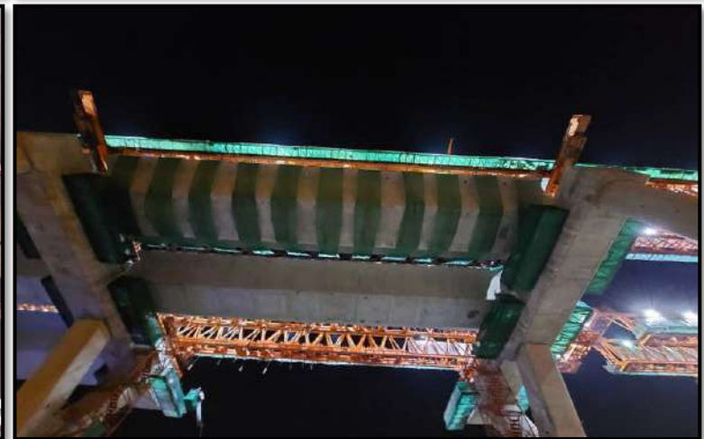
MLP03-19 to MLP03-20 Erection Segment Span (LG3)
