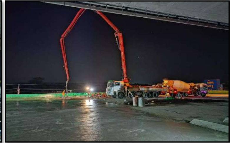
MLP01-08 to MLP01-09 Pouring Concrete Deck Slab
