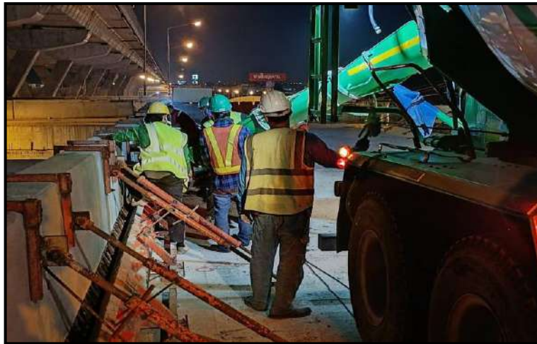
MLP01-02 to MLP01-04 Infill Concrete Precast Edge Parapet
