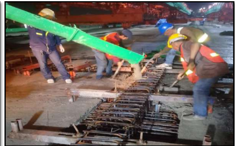
MLP03-23 to MLP03-24 Pouring Concrete Connecting Slab
