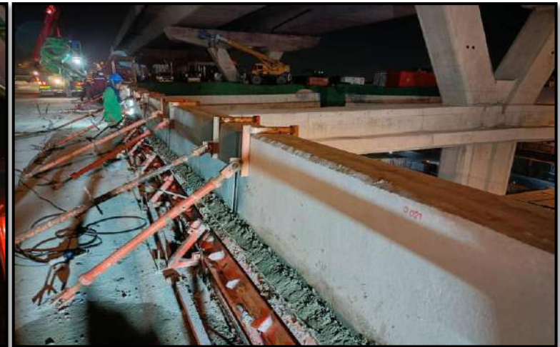
MLP01-02 to MLP01-04 Infill Concrete Precast Edge Parapet
