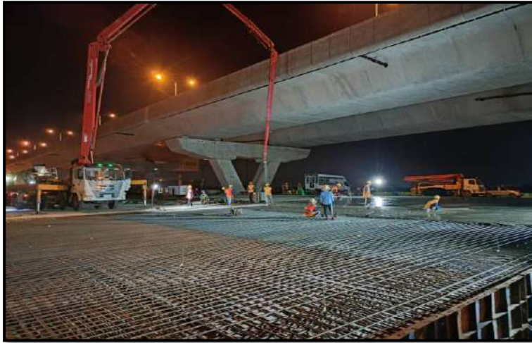
MLP01-08 to MLP01-09 Pouring Concrete Deck Slab
