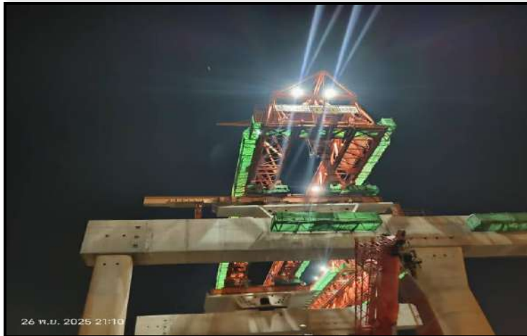
MLP03-14 Prepare Launching truss to span (LG1)
