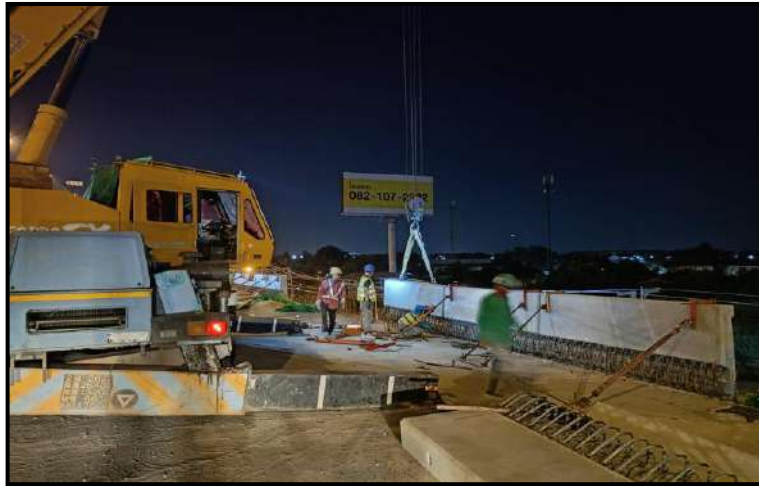
MLP01-03 to MLP01-04 Install Precast Edge Parapet
