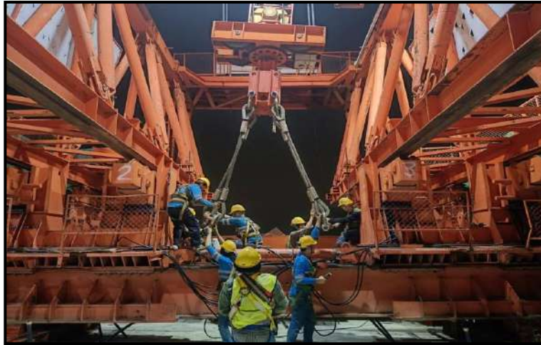
MLP03-19 Launching Gantry to Span
