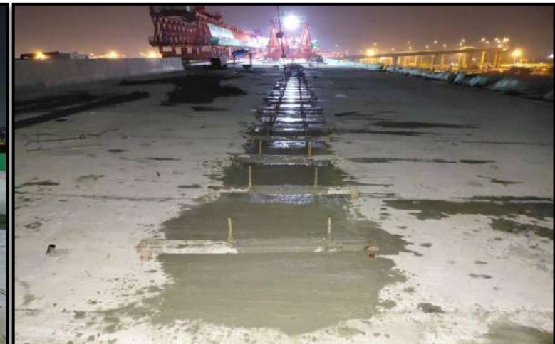
MLP03-22 to MLP03-23 Pouring Concrete Connecting Slab
