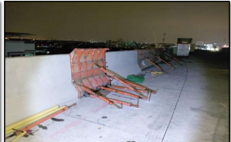
ROF2-03 to ROF2-07 Pouring Concrete Edge Parapet
