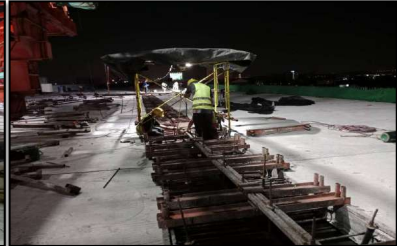
MLP03-21 to MLP03-22 Install Bottom Formwork Connecting Slab
