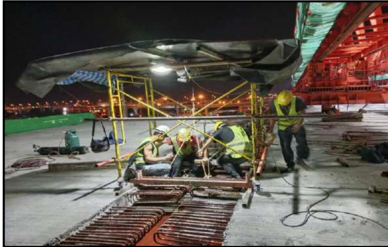
MLP03-21 to MLP03-22 Install Bottom Formwork Connecting Slab
