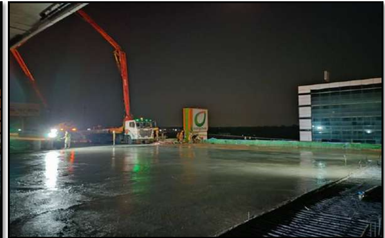
MLP01-09 to MLP01-10 Pouring Concrete Deck Slab
