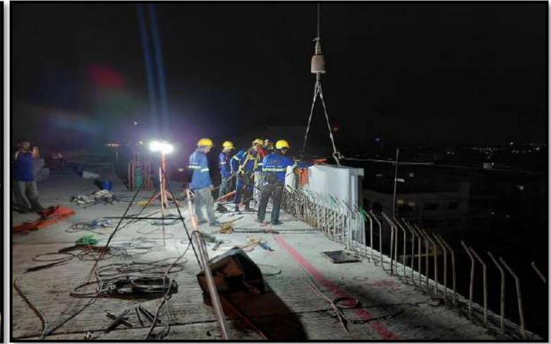
MLP03-22 to MLP03-23 Install Precast Edge Parapet
