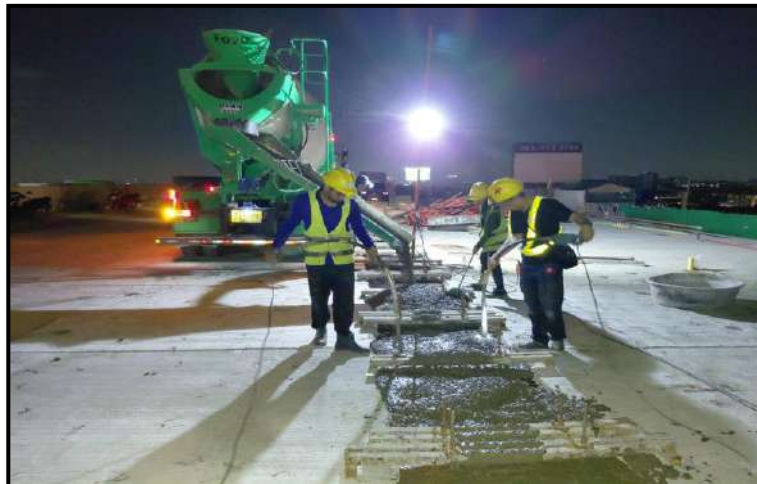
MLP03-22 to MLP03-23 Pouring Concrete Connecting Slab
