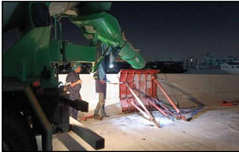
ROF2-03 to ROF2-07 Pouring Concrete Edge Parapet
