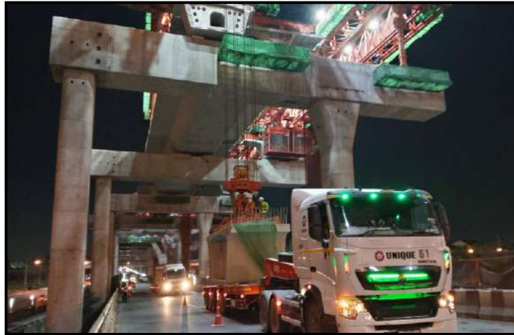
MLP03-12 to MLP03-13 Install Precast Segment
