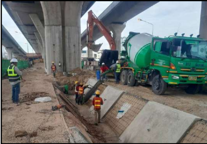
Pouring Concrete Lining Ditch MLP01-21C to MLP01-22C
