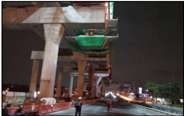
MLP03-19 to MLP03-20 Install Precast Segment
