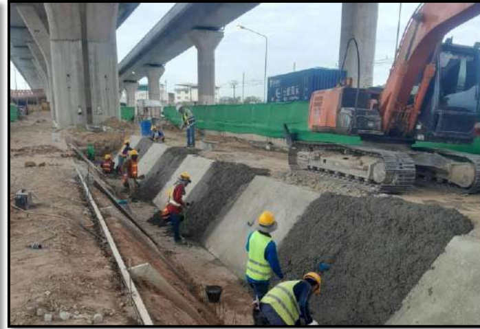
Pouring Concrete Lining Ditch MLP01-21C to MLP01-22C
