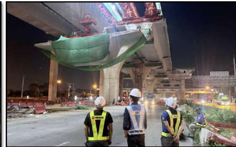
MLP03-18 to MLP03-19 Install Precast Segment
