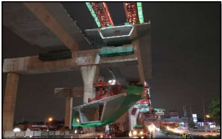
MLP03-19 to MLP03-20 Install Precast Segment
