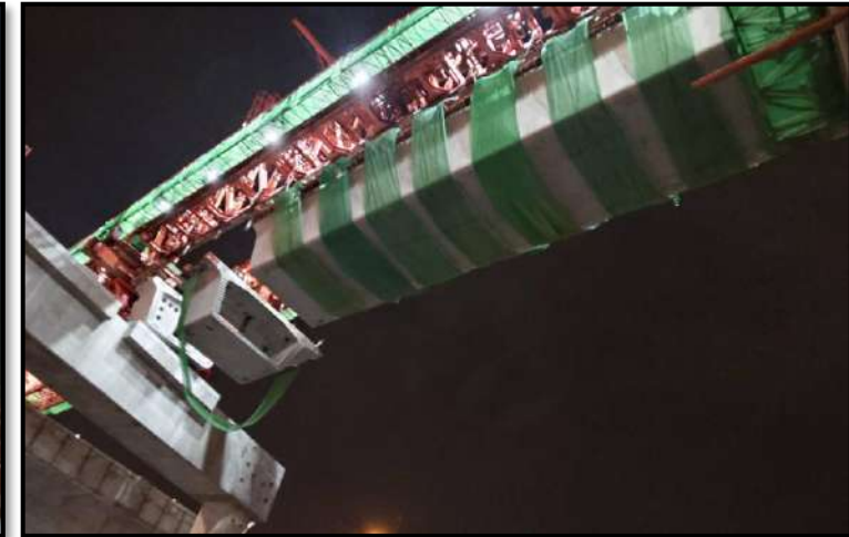
MLP03-12 to MLP03-13 Install Precast Segment
