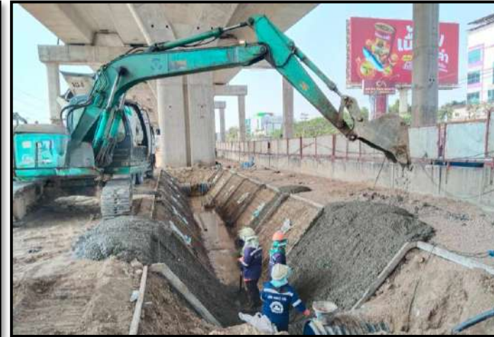
Pouring Concrete Lining Ditch MLP04-05C to MLP04-06C
