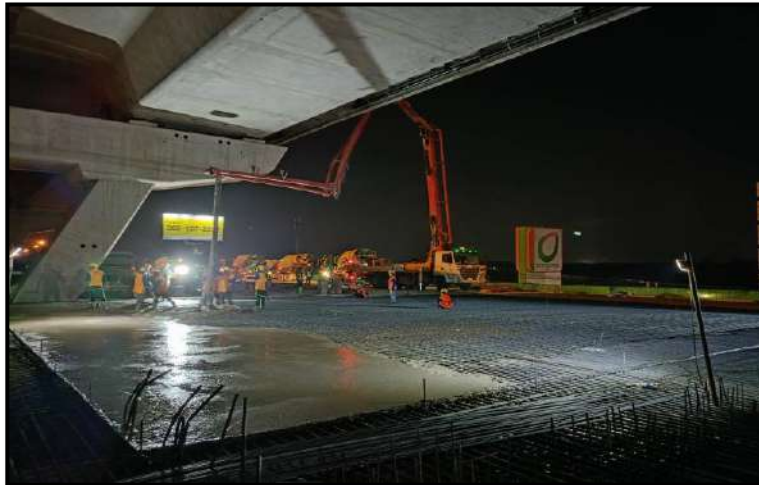
MLP01-09 to MLP01-10 Pouring Concrete Deck Slab
