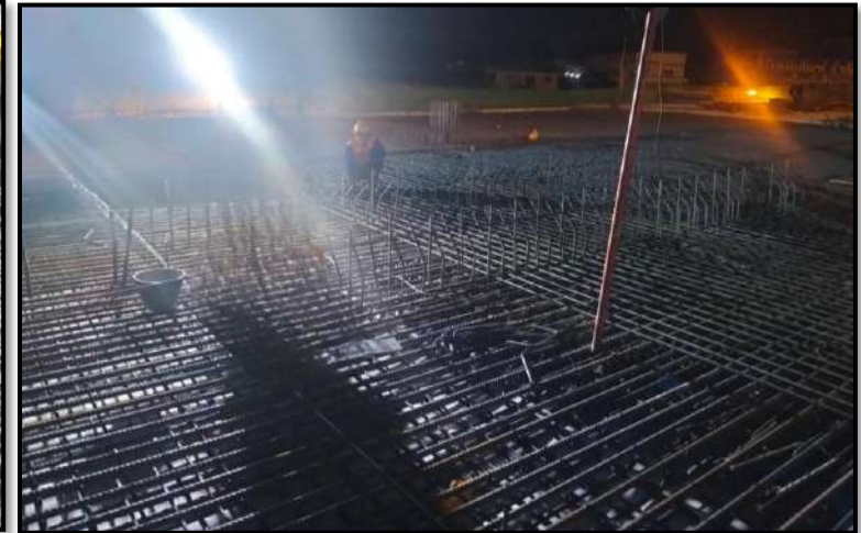
MLP01-09 to MLP01-10 Install Reinforcement Deck Slab
