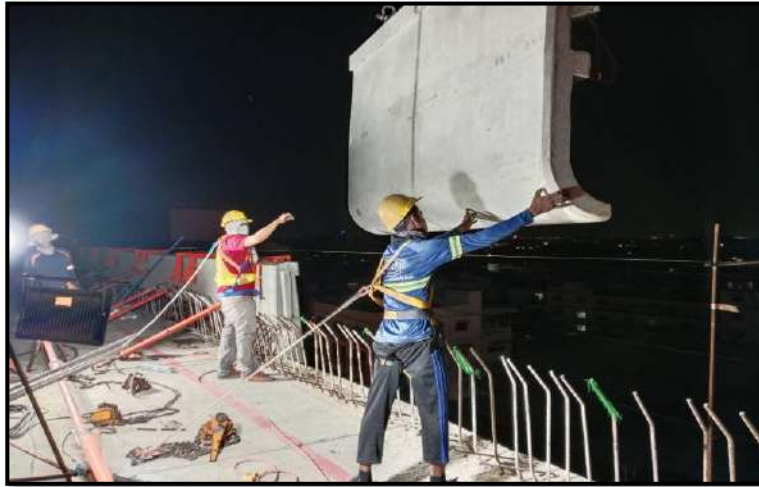
MLP03-22 to MLP03-23 Install Precast Edge Parapet
