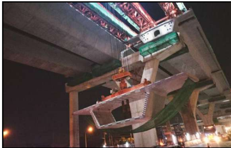
MLP03-18 to MLP03-19 Install Precast Segment
