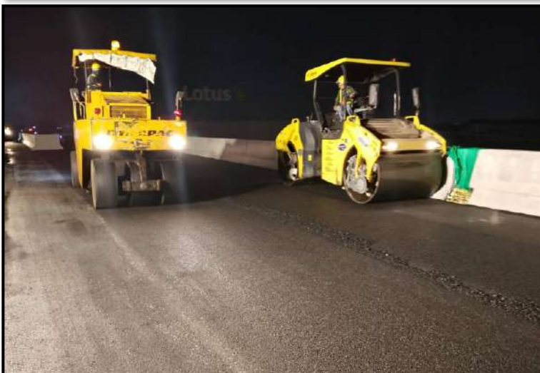
Asphaltic Concrete Pavement (Zone2)
