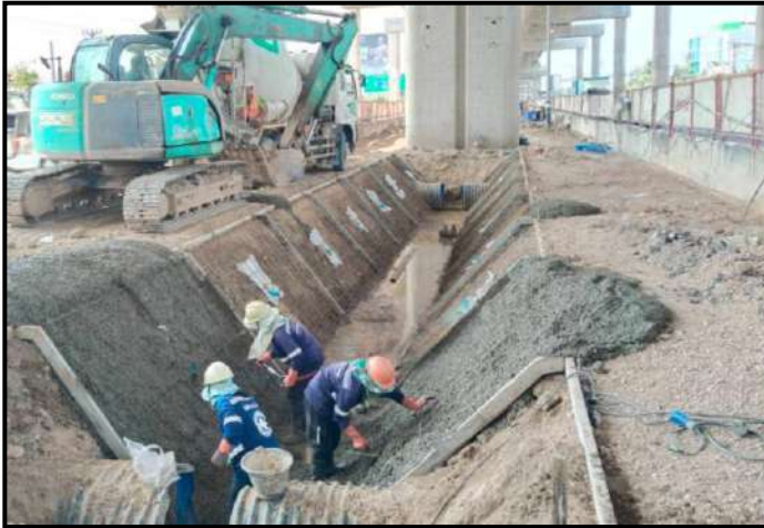
Pouring Concrete Lining Ditch MLP04-05C to MLP04-06C
