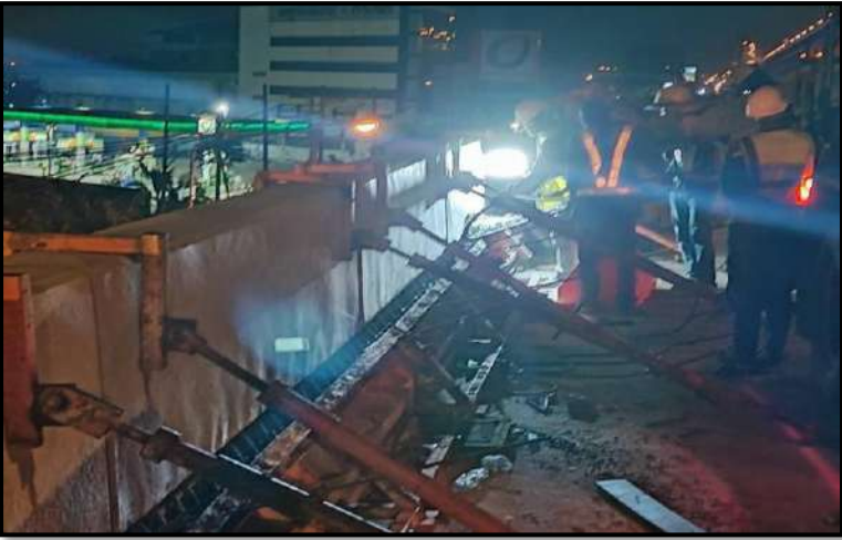
MLP01-03 to MLP01-04 Infill Concrete Precast Edge Parapet
