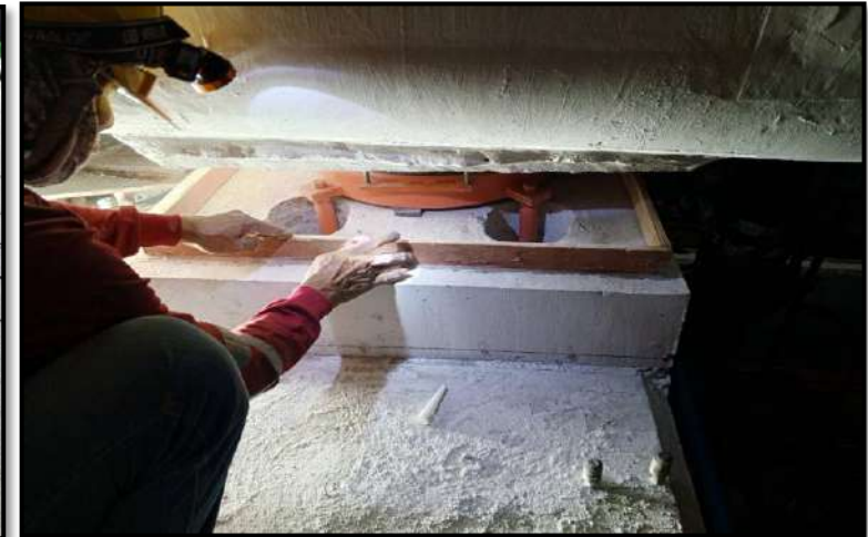
MLP03-15 Grout Top Pot Bearing (LG1)
