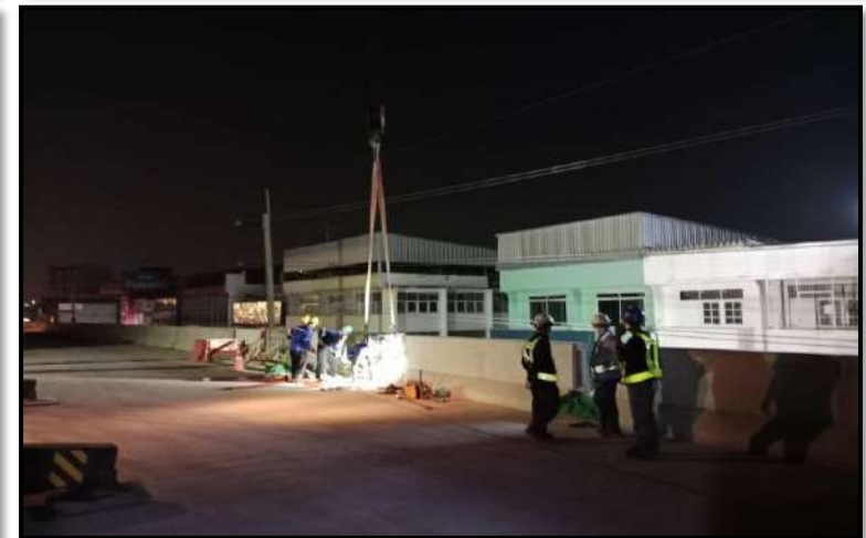
RON2-18 to MLP04-15 Install Precast Edge Parapet
