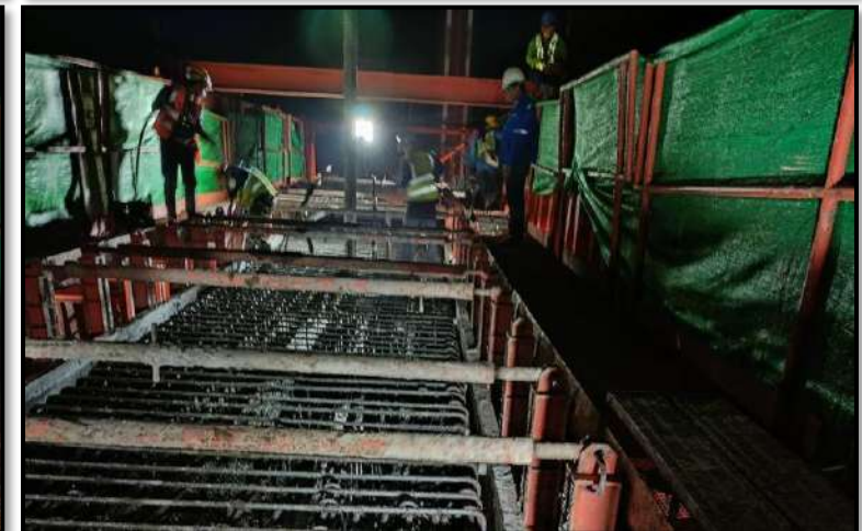
MLP01-13 Pouring Concrete Lower Crossbeam Type YT-1 Step 1
