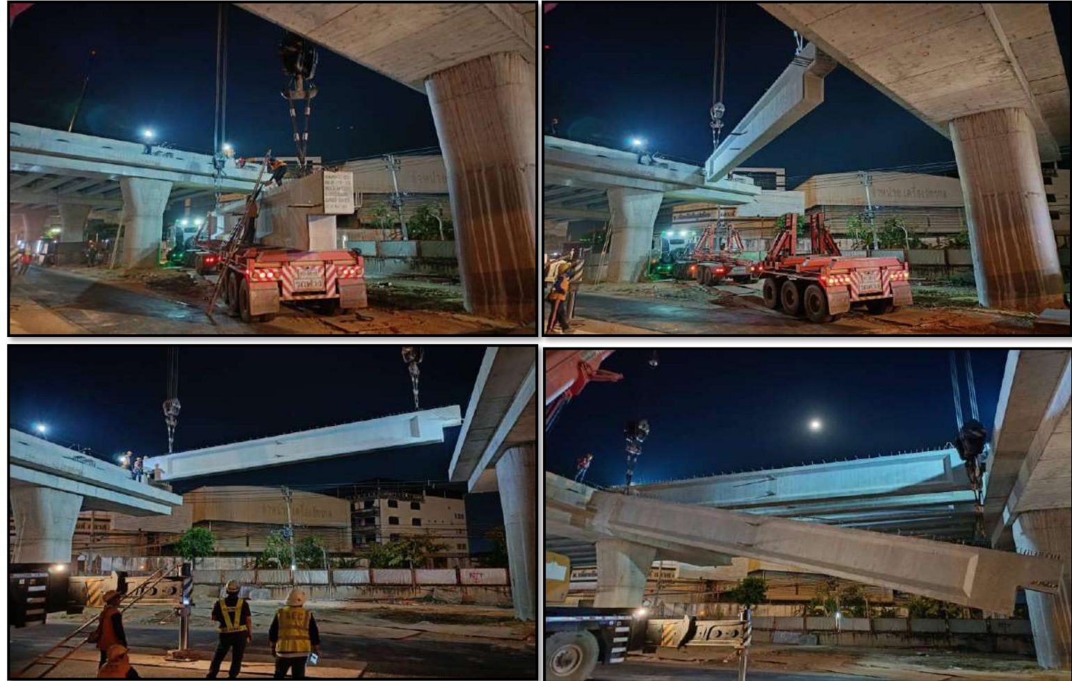
MLP01-12 to MLP01-13 Install Precast I-Girder
