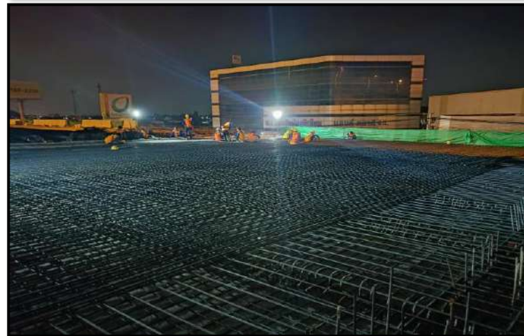
MLP01-11 to MLP01-12 Install Reinforcement Deck Slab
