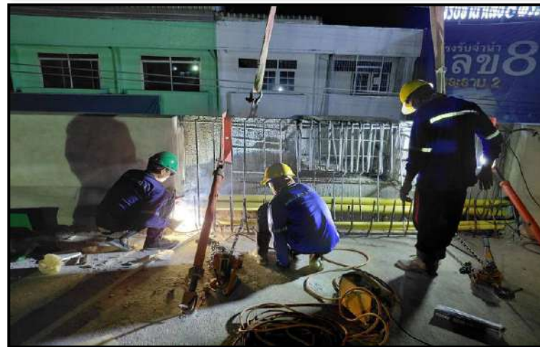
RON2-18 to MLP04-15 Install Precast Edge Parapet
