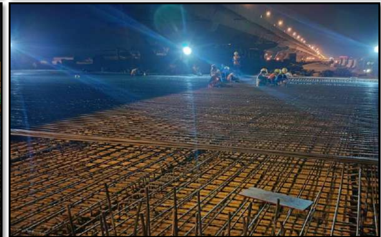
MLP01-11 to MLP01-12 Install Reinforcement Deck Slab
