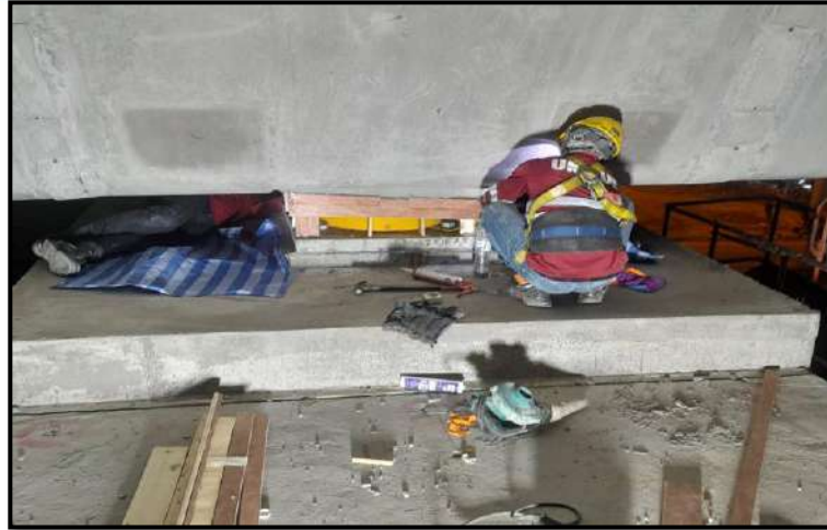
MLP03-14 Install Form Work Top Pot Bearing Pier (LG2)
