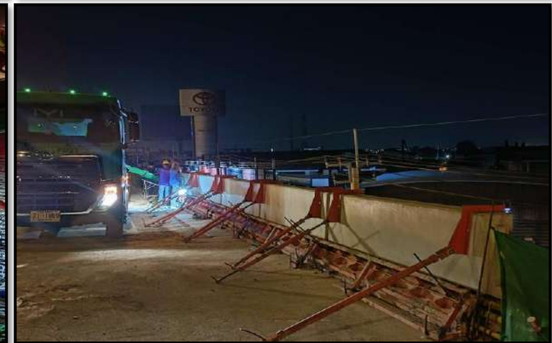
MLP01-10 to MLP01-11 Infill Concrete Precast Edge Parapet
