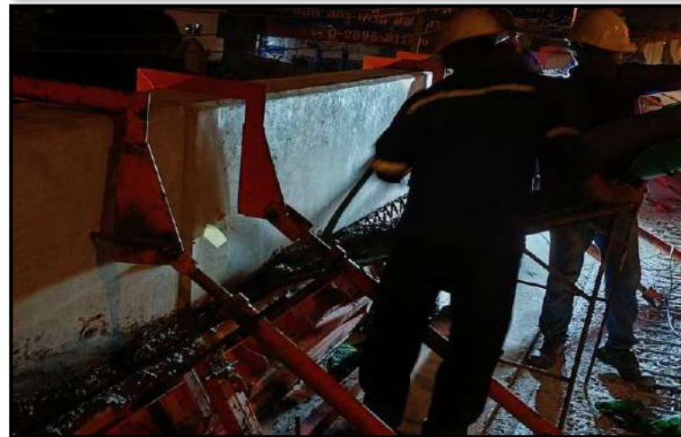
MLP01-10 to MLP01-11 Infill Concrete Precast Edge Parapet
