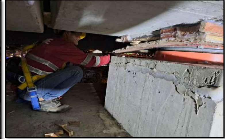
MLP03-14 Install Form Work Top Pot Bearing Pier (LG2)
