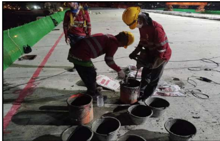
MLP03-15 Grout Top Pot Bearing (LG1)
