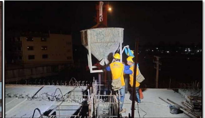
MLP01-13 to MLP01-14 Pouring Concrete Girder Diaphragm
