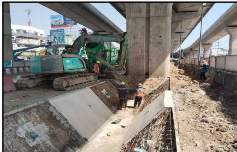
MLP04-07C to MLP04-08C Pouring Concrete Wall of Lining Ditch
