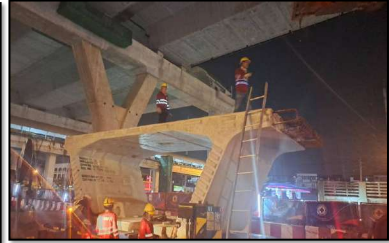
MLP03-13 to MLP03-14 Install Precast Segment (LG2)
