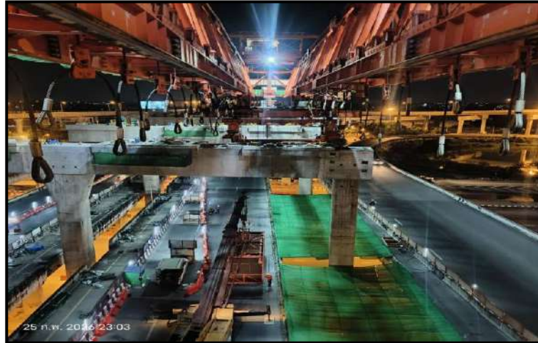
MLP03-09 Install Precast Segment (LG1)
