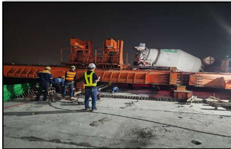
MLP03-20 Pouring Concrete Connecting Slab
