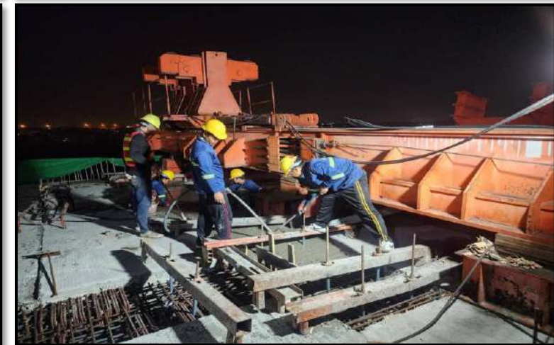
MLP03-20 Pouring Concrete Connecting Slab
