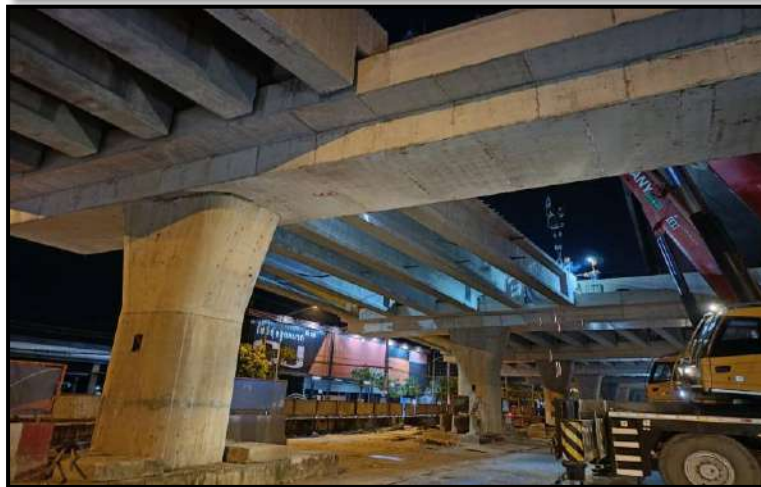
MLP01-12 to MLP01-13 Install Precast I-Girder
