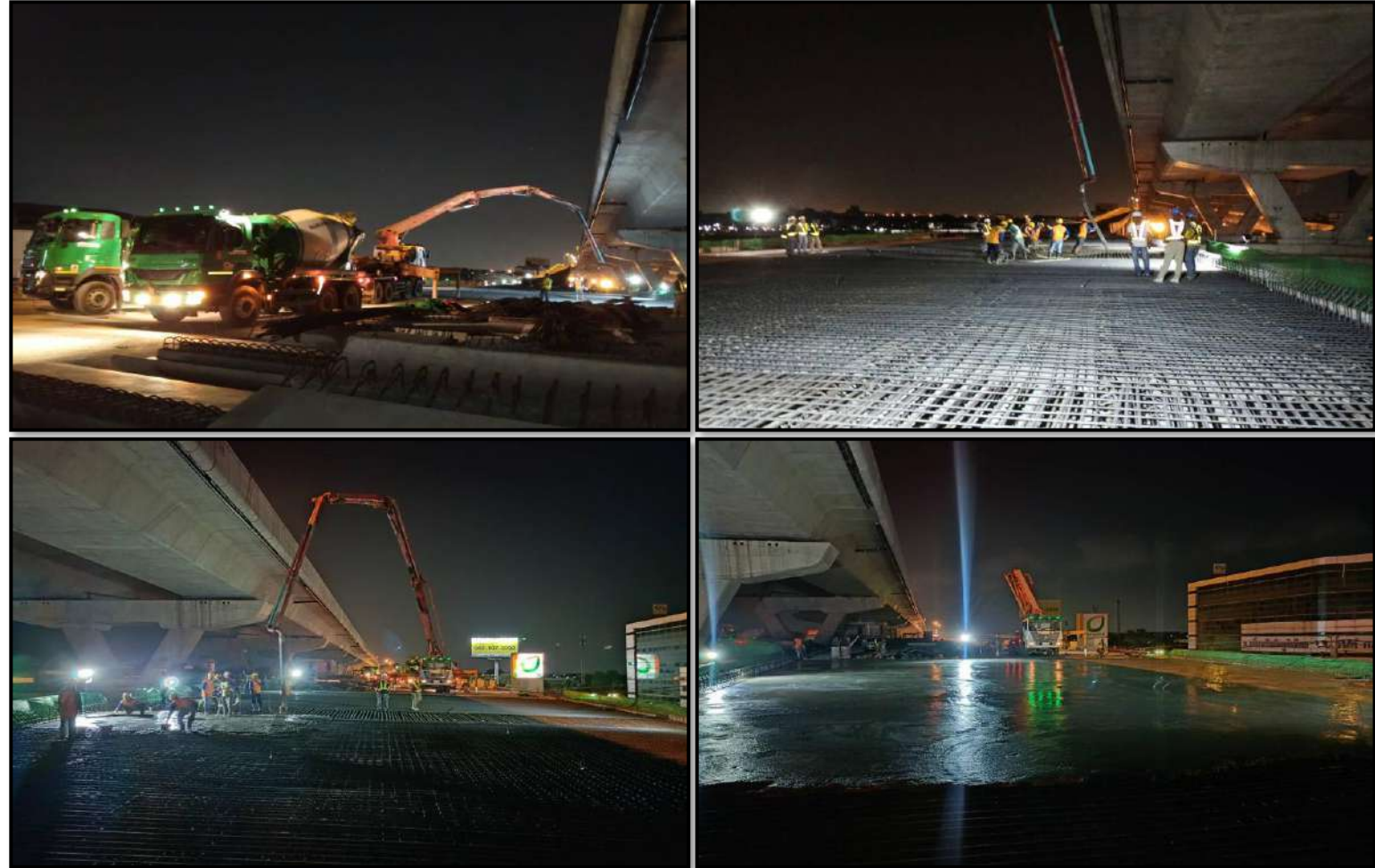
MLP01-11 to MLP01-12 Pouring Concrete Deck Slab
