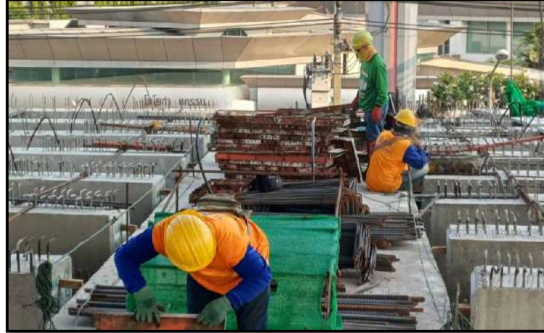
MLP01-13 to MLP01-14 Install Reinforcement and Formwork Girder Diaphragm
