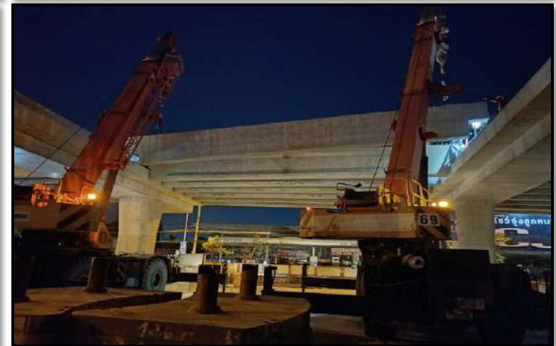
MLP01-12 to MLP01-13 Install Precast I-Girder
