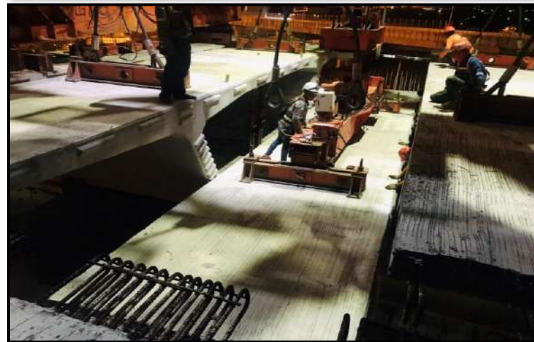
MLP03-01 to MLP03-02 Install Precast Segment (LG6)
