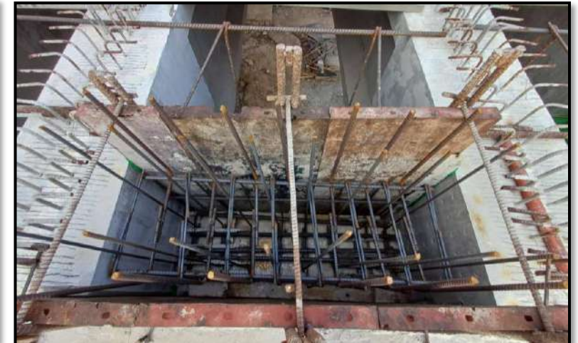
MLP01-13 to MLP01-14 Install Reinforcement and Formwork Girder Diaphragm
