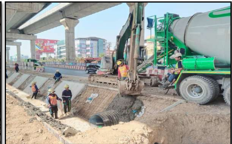
MLP04-07C to MLP04-08C Pouring Concrete Wall of Lining Ditch
