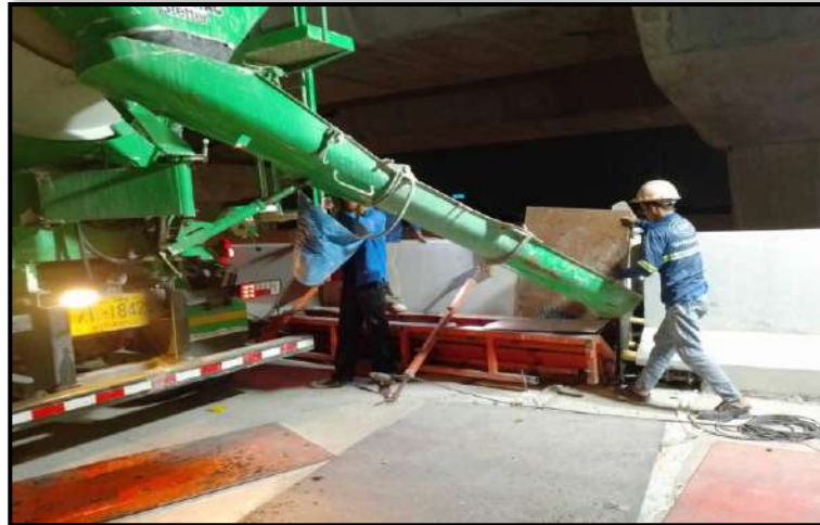
ROF2-03 to ROF2-07 Pouring Concrete Edge Parapet
