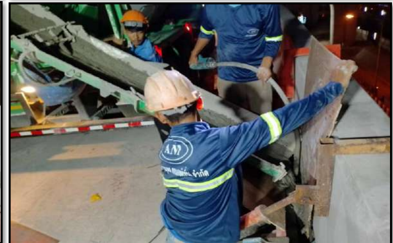
ROF2-03 to ROF2-07 Pouring Concrete Edge Parapet
