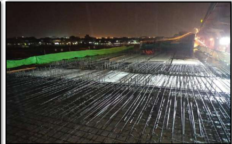
MLP01-13 to MLP01-14 Install Reinforcement Deck Slab
