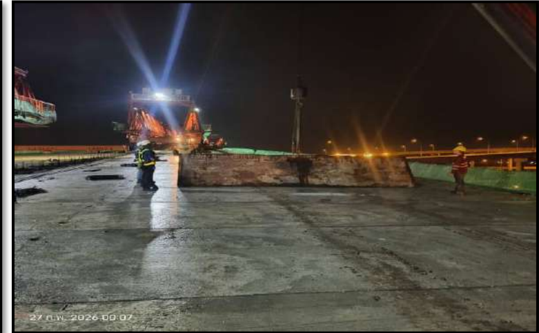
MLP03-09 Install Precast Segment (LG1)
