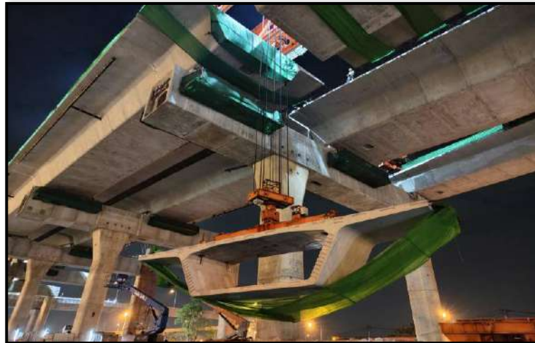
MLP03-17 to MLP03-18 Install Precast Segment (LG4)
