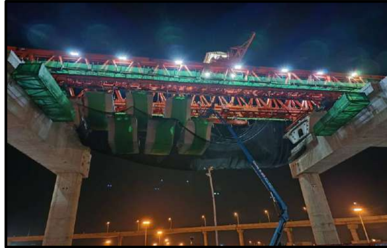
MLP03-09 to MLP03-08 Install Precast Segment (LG1)
