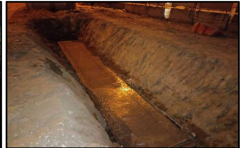
MLP01-09 to MLP01-12 Pouring Concrete Slab of Lining Ditch
