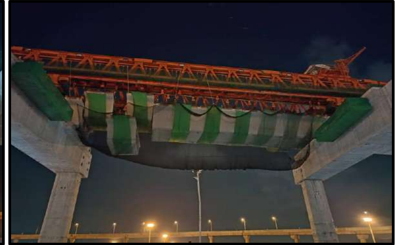
MLP03-09 to MLP03-08 Install Precast Segment (LG1)
