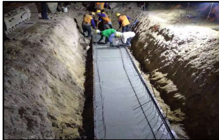
MLP01-09 to MLP01-12 Pouring Concrete Slab of Lining Ditch
