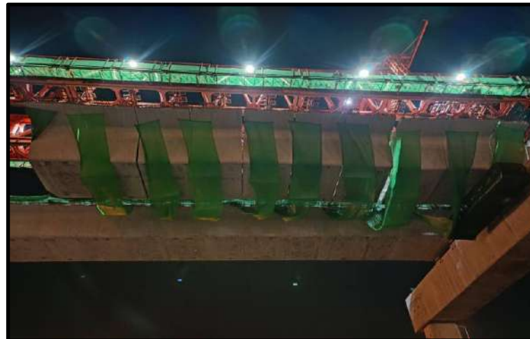
MLP03-11 to MLP03-12 Install Precast Segment (LG2)
