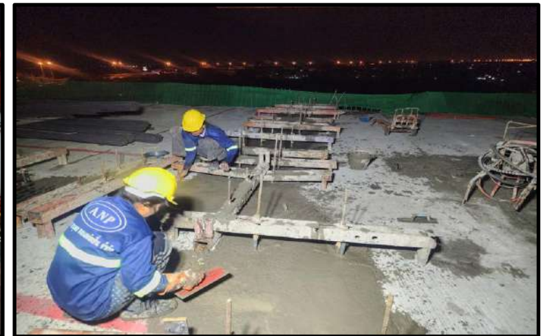
MLP03-18 Pouring Concrete Connecting Slab
