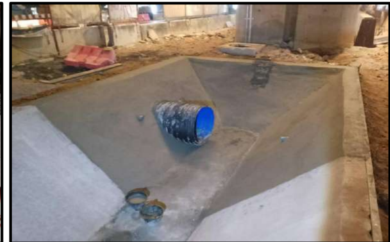
MLP04-15 Pouring Concrete Wall of Lining Ditch
