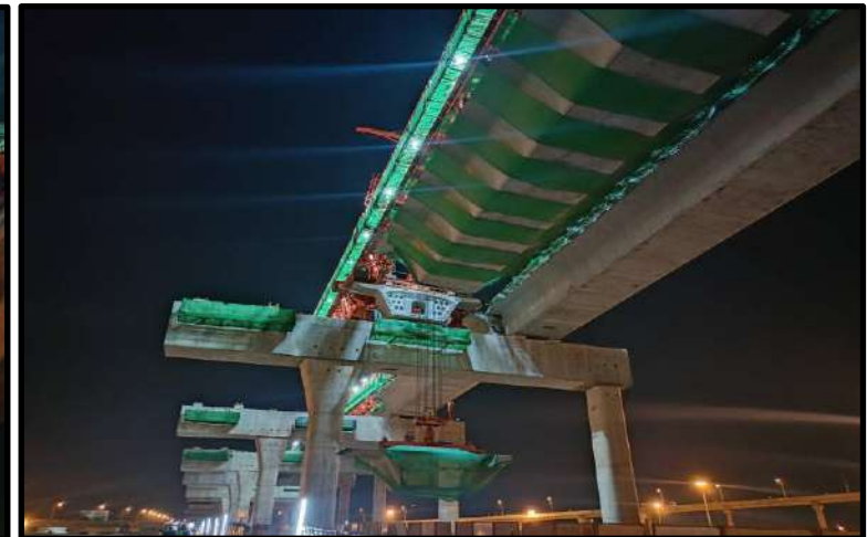
MLP03-11 to MLP03-12 Install Precast Segment (LG2)
