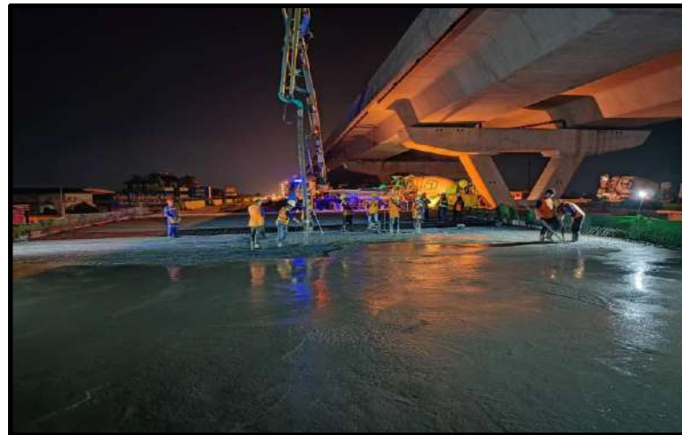
MLP01-11 to MLP01-13 Pouring Concrete Deck Slab
