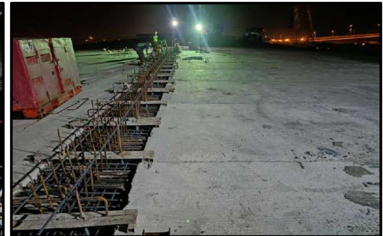
MLP03-17 to MLP03-18 Install Reinforcement Connecting Slab
