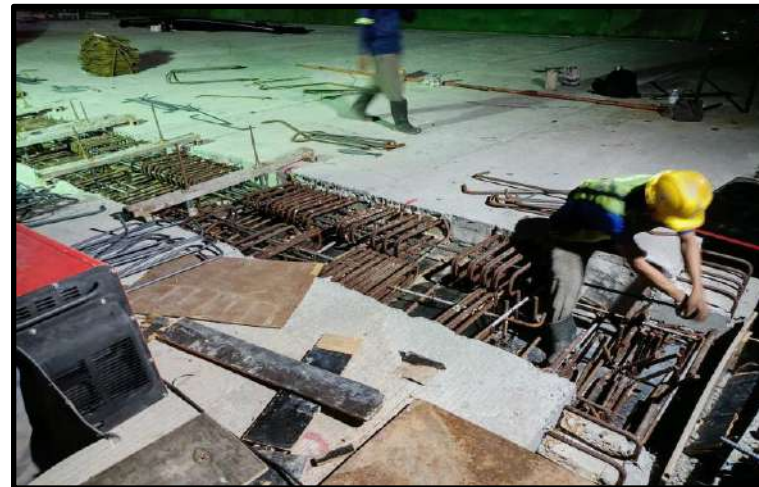
MLP03-17 to MLP03-18 Install Reinforcement Connecting Slab
