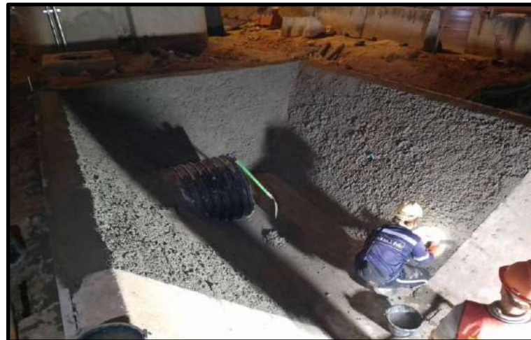
MLP04-15 Pouring Concrete Wall of Lining Ditch
