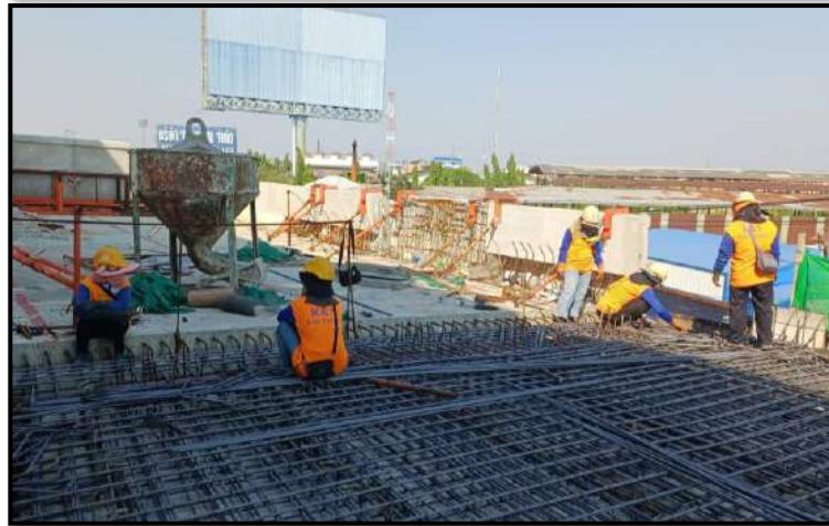
MLP01-13 to MLP01-14 Install Reinforcement Deck Slab
