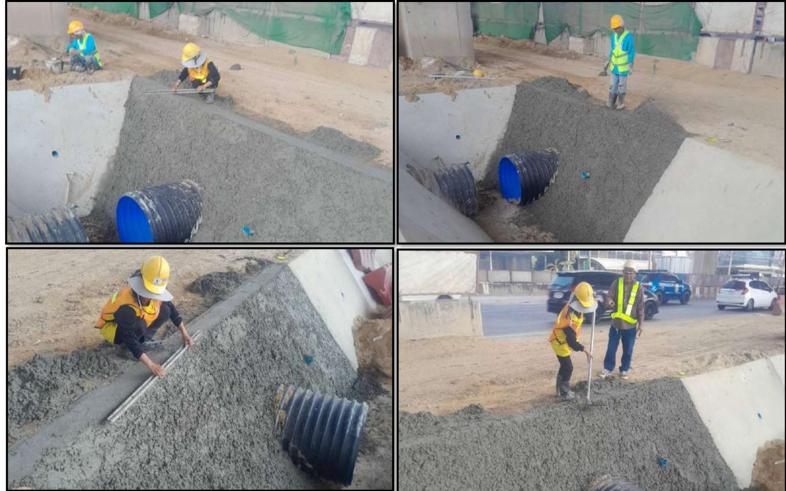
MLP01-24C Pouring Concrete Wall of Lining Ditch
