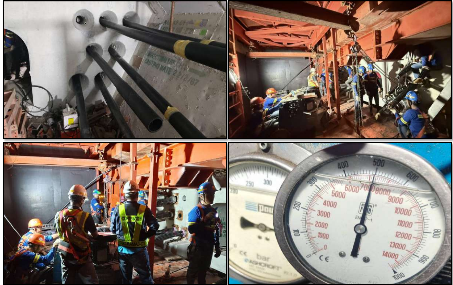
MLP03-07 to MLP03-08 Stressing Tendon Precast Segment
