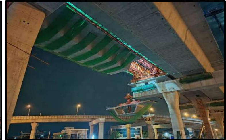
MLP03-02 to MLP03-03 Install Precast Segment (LG6)
