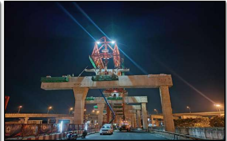
MLP03-05 Install Precast Pier Segment (LG5)
