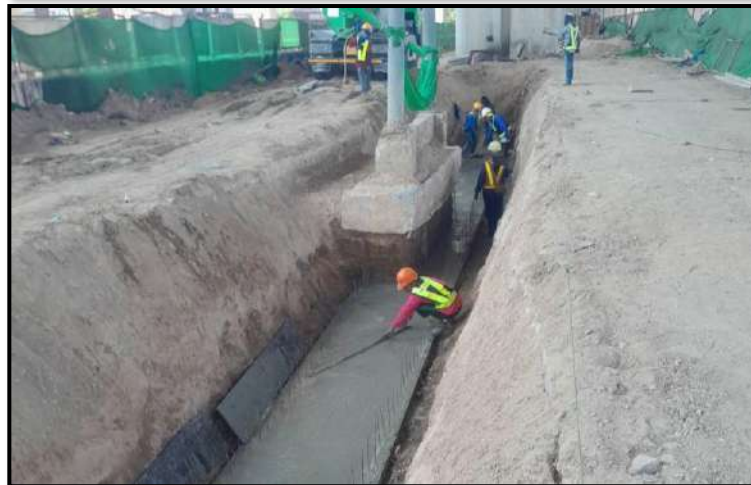
MLP02-13C to MLP02-14C Pouring Concrete Slab of Lining Ditch
