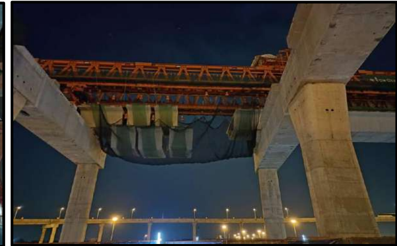
MLP03-06 to MLP03-07 Install Precast Segment (LG1)
