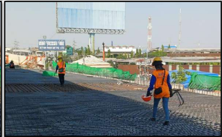
MLP01-13 to MLP01-14 Install Reinforcement Deck Slab
