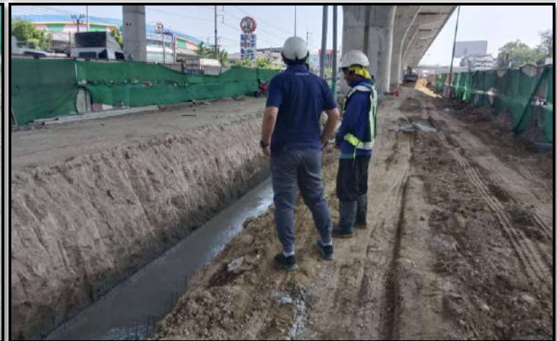
MLP02-13C to MLP02-14C Pouring Concrete Slab of Lining Ditch
