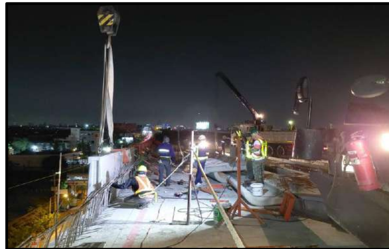
MLP03-17LT to MLP03-21LT Install Precast Edge Parapet
