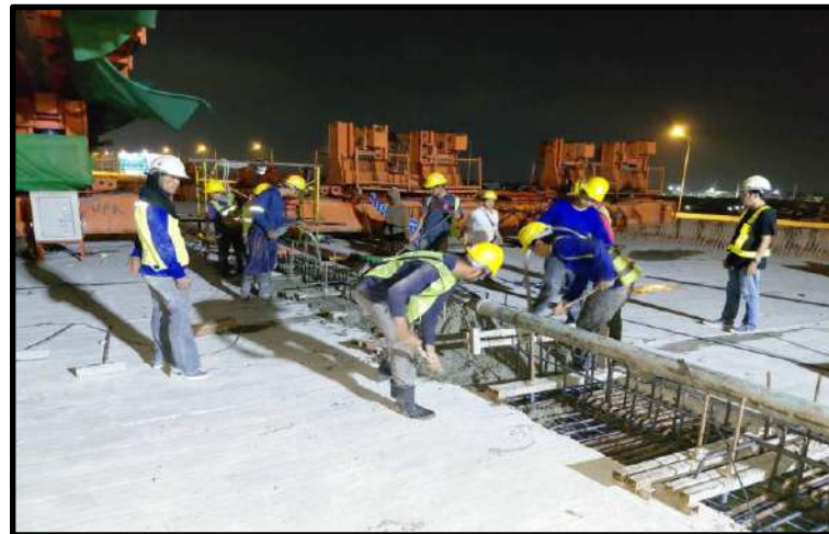
MLP02-26 to MLP03-02 Pouring Concrete Connecting Slab
