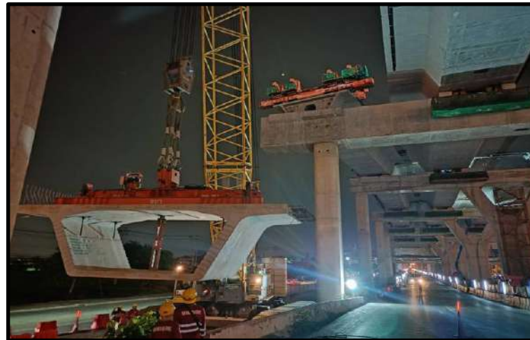
MLP03-06 to MLP03-07 Install Precast Segment (LG1)
