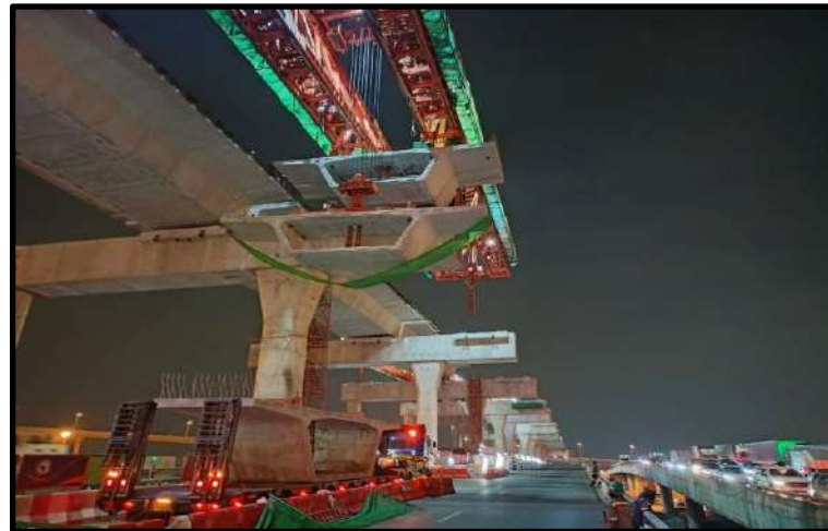
MLP03-02 to MLP03-03 Install Precast Segment (LG6)
