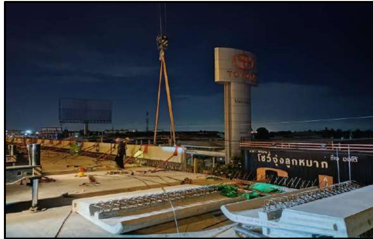
MLP01-11RT to MLP01-12RT Install Precast Edge Parapet
