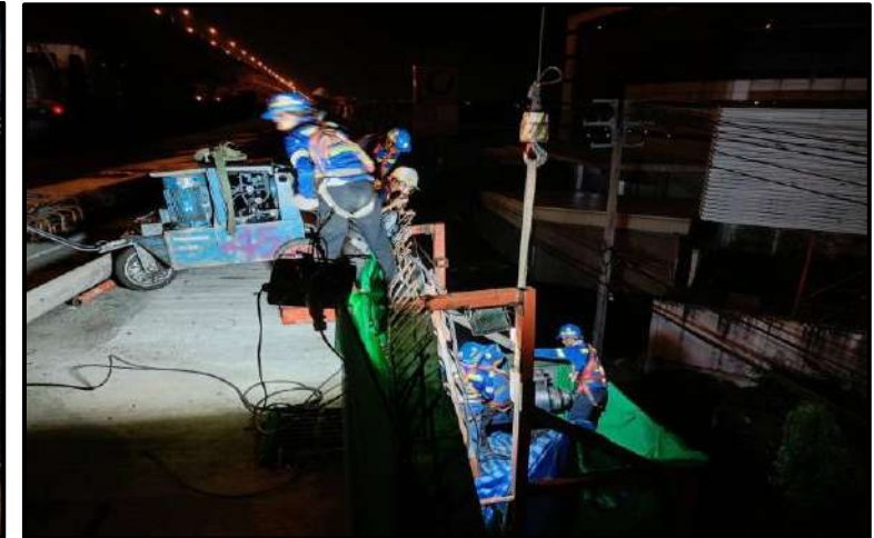
MLP01-12 Stressing Tendon Lower Crossbeam Type PTT-1
