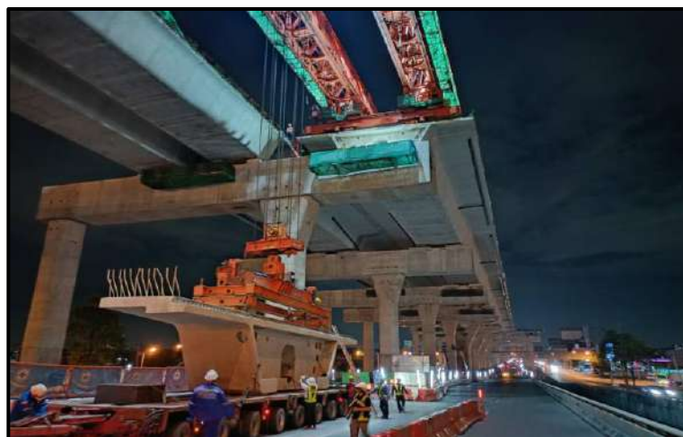
MLP03-13 to MLP03-14 Install Precast Segment (LG2)
