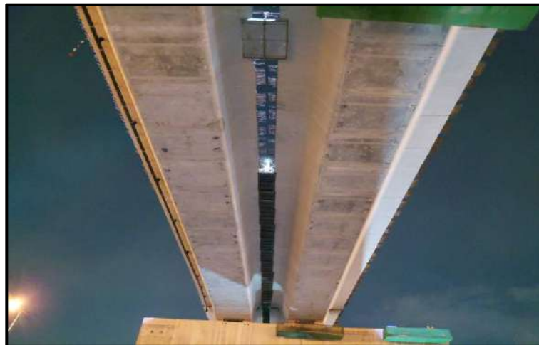
MLP03-11 to MLP03-14 Install Bottom Formwork Connecting Slab
