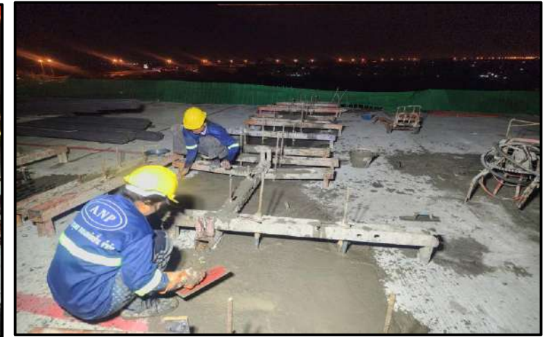
MLP03-18 Pouring Concrete Connecting Slab
