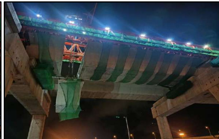
MLP03-08 to MLP03-09 Install Precast Segment (LG1)
