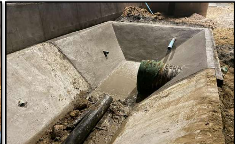
MLP04-22C to MLP04-23C Pouring Concrete Wall of Lining Ditch
