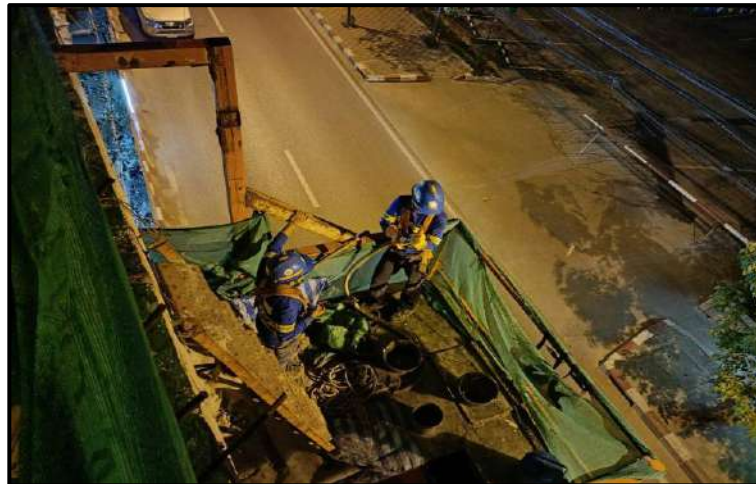
MLP01-13 Grouting Tendon Lower Crossbeam Type YT-1
