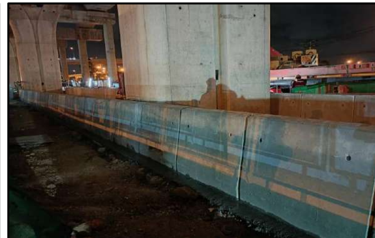
MLP03-19 to MLP03-22 Pouring Concrete Locking Barrier Single Slope
