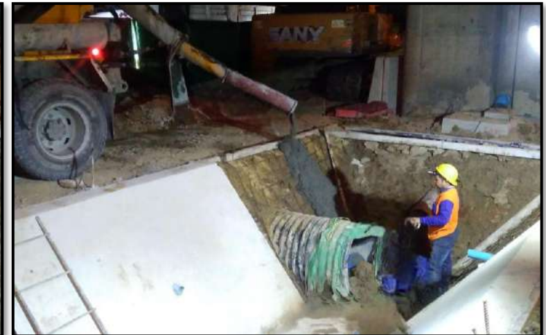
MLP01-15C to MLP01-16C Pouring Concrete Wall of Lining Ditch
