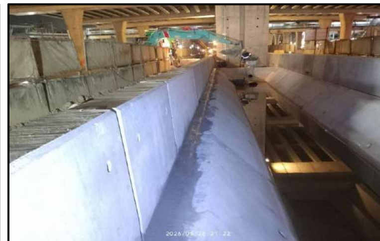
MLP04-14 to MLP04-15 Pouring Concrete Locking Barrier Single Slope
