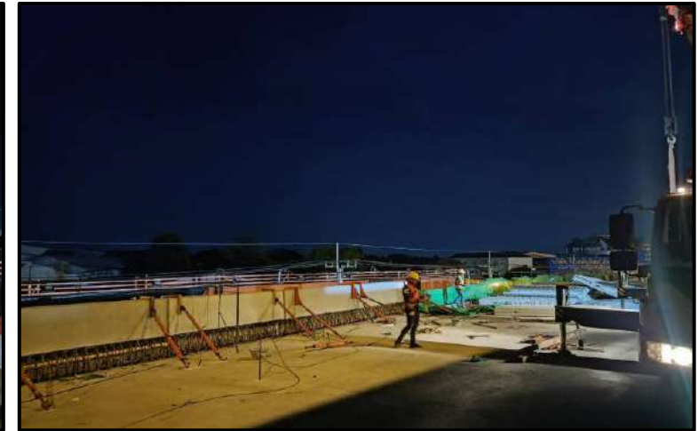
MLP01-11RT to MLP01-12RT Install Precast Edge Parapet
