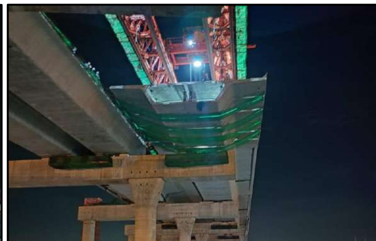
MLP03-13 to MLP03-14 Install Precast Segment (LG2)
