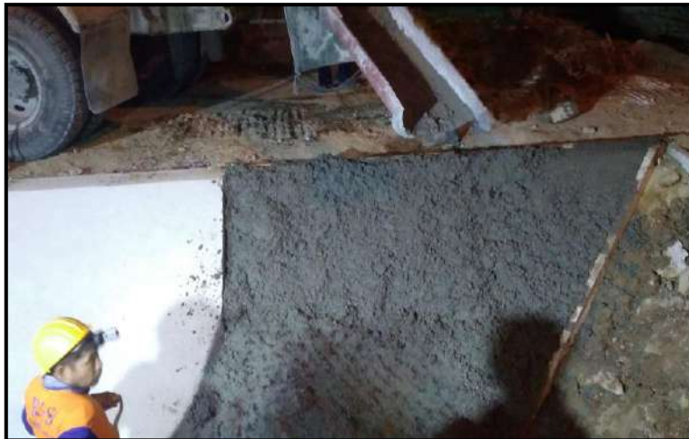
MLP01-15C to MLP01-16C Pouring Concrete Wall of Lining Ditch
