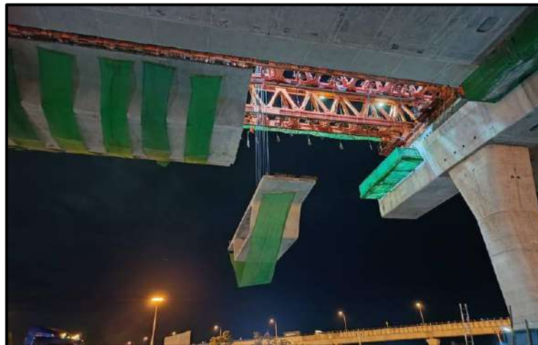
MLP03-04 to MLP03-05 Install Precast Segment (LG6)
