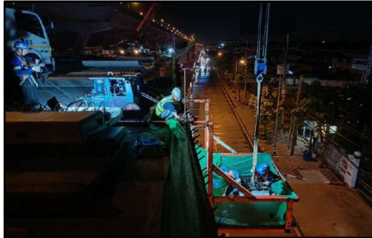
MLP01-12 Stressing Tendon Lower Crossbeam Type PTT-1
