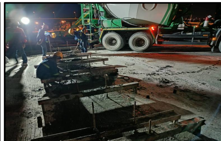
MLP03-08 Pouring Concrete Connecting Slab
