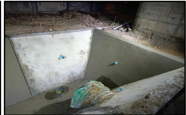
MLP01-09C to MLP01-11C Pouring Concrete Wall of Lining Ditch
