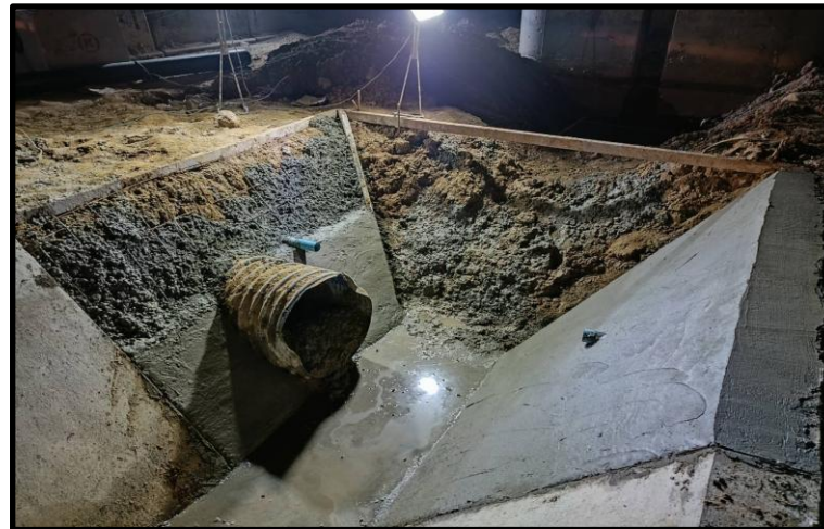
MLP01-09C to MLP01-11C Pouring Concrete Wall of Lining Ditch
