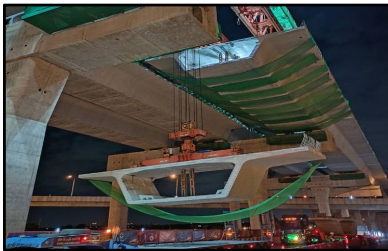
MLP03-10 to MLP03-11 Install Precast Segment (LG2)
