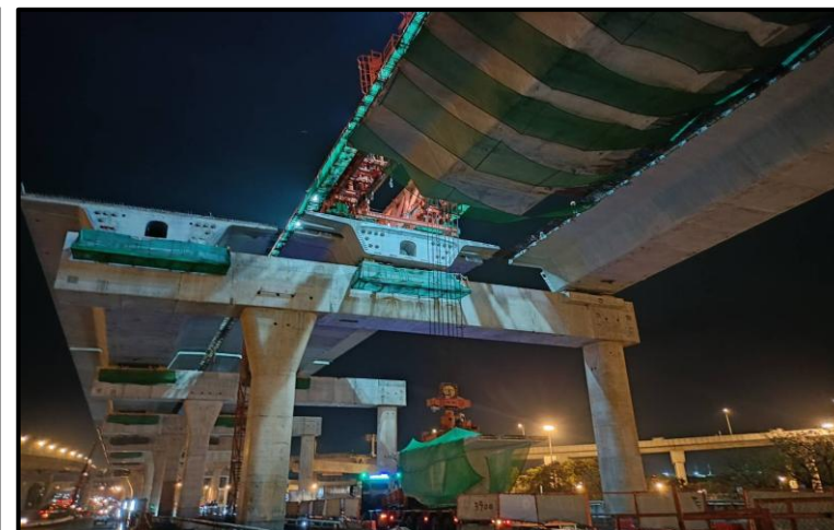
MLP03-05 to MLP03-06 Install Precast Segment (LG1)
