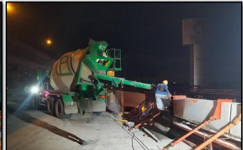
MLP01-11RT, MLP01-12RT Infill Concrete Precast Edge Parapet
