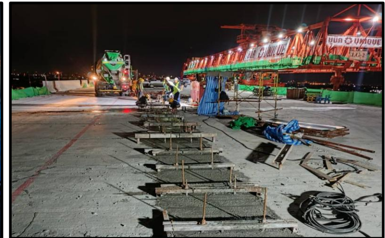
MLP03-08 to MLP03-09 Pouring Concrete Connecting Slab
