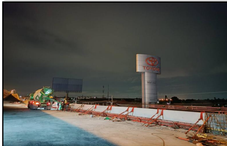
MLP01-11RT, MLP01-12RT Infill Concrete Precast Edge Parapet
