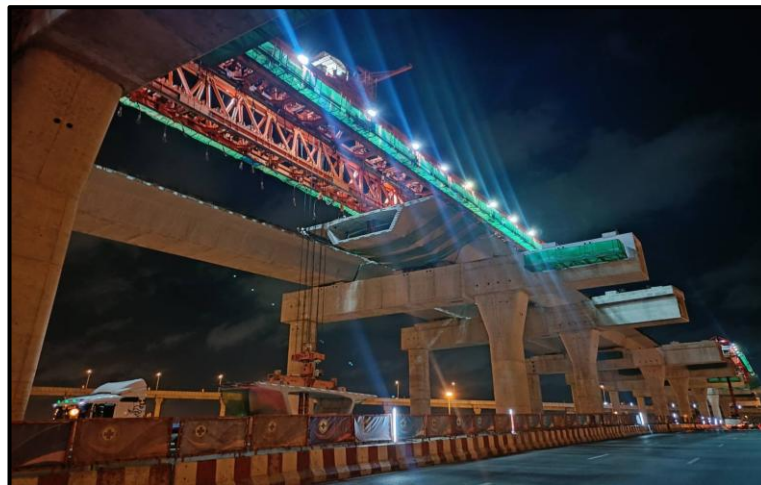
MLP03-05 to MLP03-06 Install Precast Segment (LG1)
