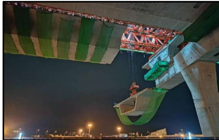
MLP03-09 to MLP03-10 Install Precast Segment (LG2)
