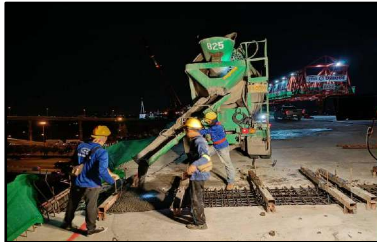
MLP03-03 & MLP03-04 Pouring Concrete Connecting Slab
