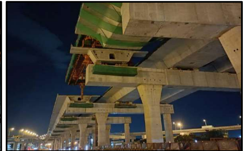
MLP03-06 to MLP03-07 Install Precast Segment (LG2)
