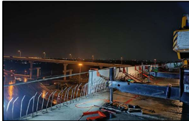
MLP03-08LT to MLP03-09LT Install Precast Edge Parapet
