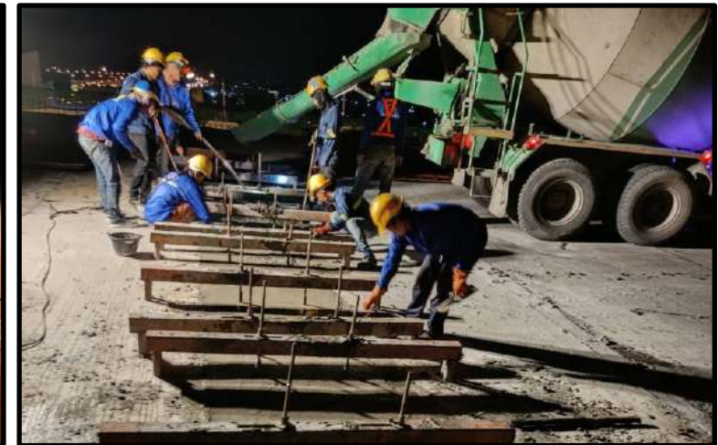
MLP03-03 & MLP03-04 Pouring Concrete Connecting Slab
