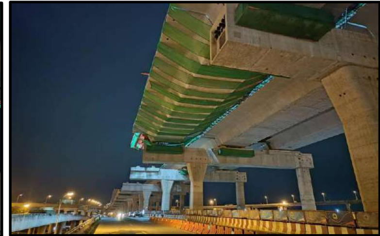
MLP03-09 to MLP03-10 Install Precast Segment (LG2)
