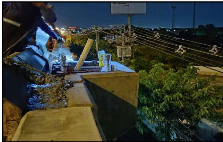
MLP01-09LT, MLP01-14LT Pouring Concrete Parapet
