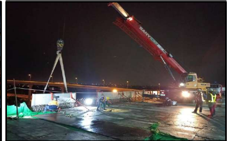
MLP03-08LT to MLP03-09LT Install Precast Edge Parapet
